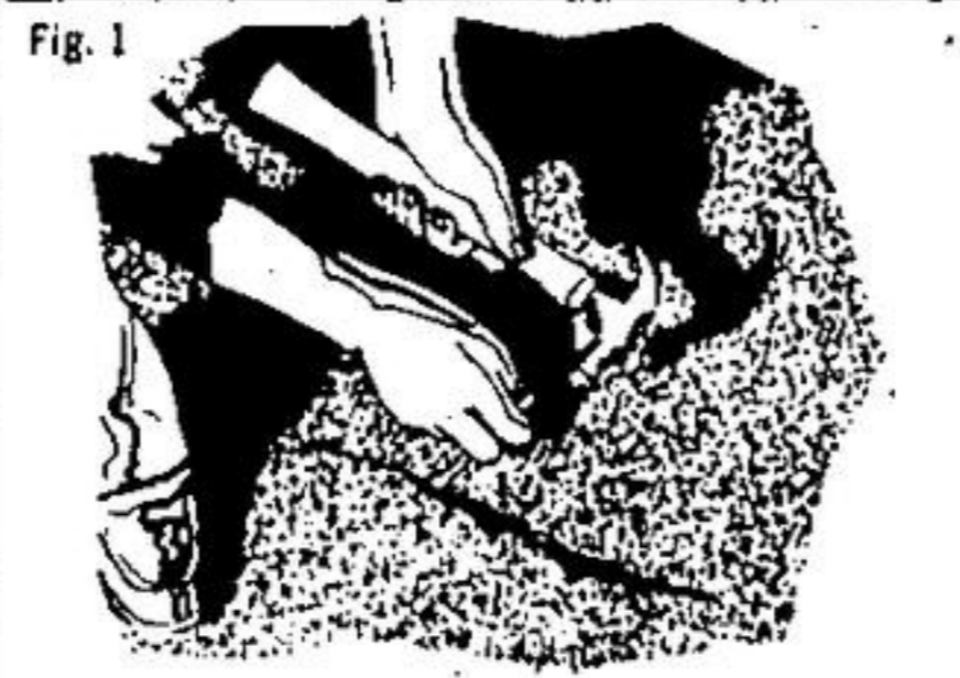
Enlarge crack with cold chisel and hammer before attempting to repair it
