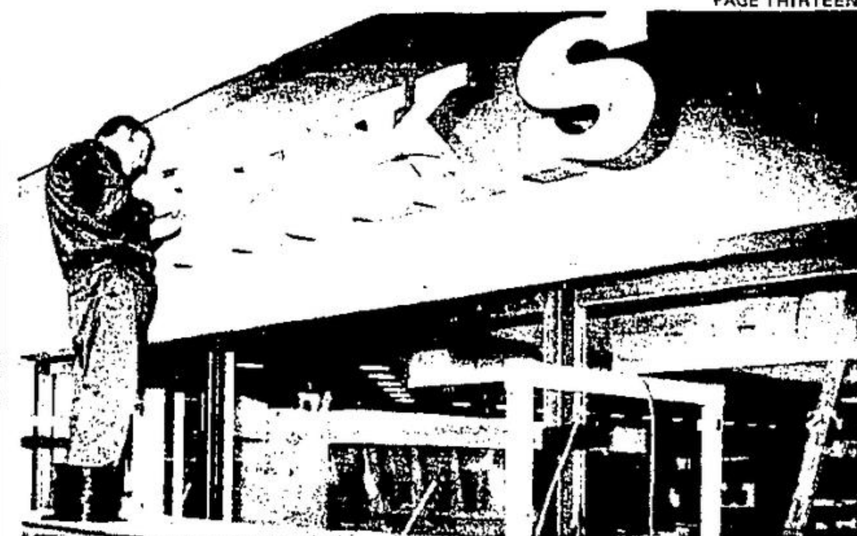
BIRKS SIGN BEING INSTALLED
