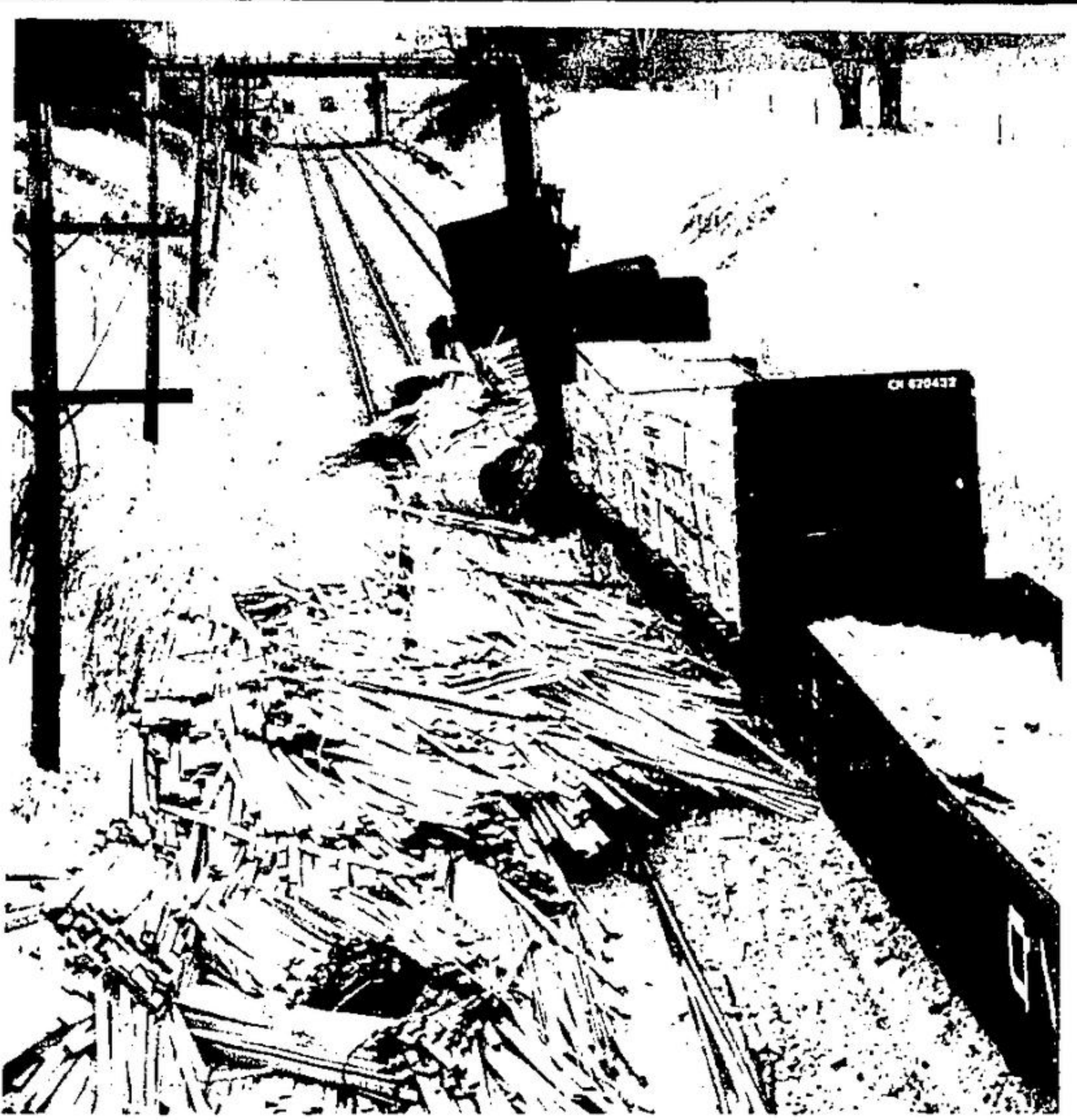
A mobile crane, a truck with railway wheels, begins to clear wreckage from the two CN tracks leading into Georgetown station. The overpass in the background is Mountainview Road.
