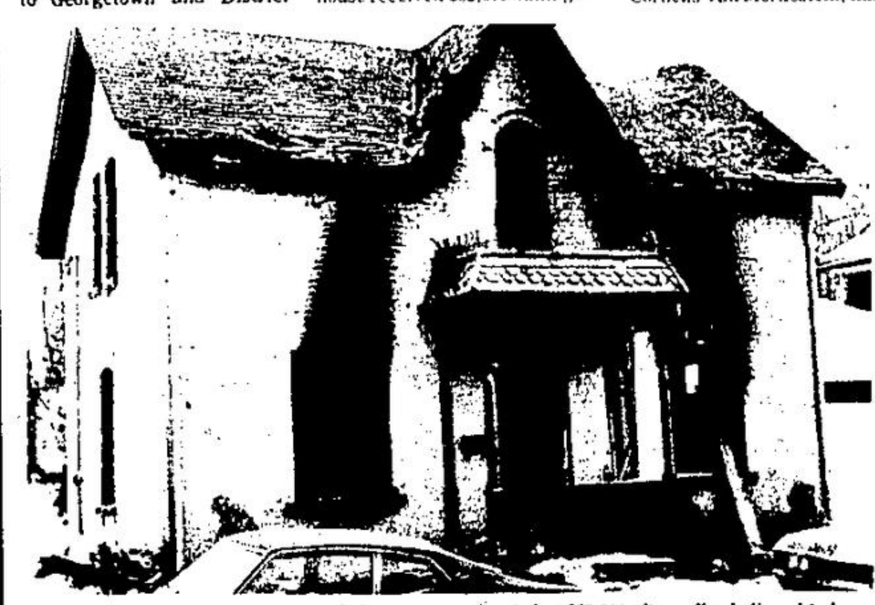
Damage to the Van Merksteijn home was estimated at $62,000 after a fire believed to have been caused by careless smoking.
