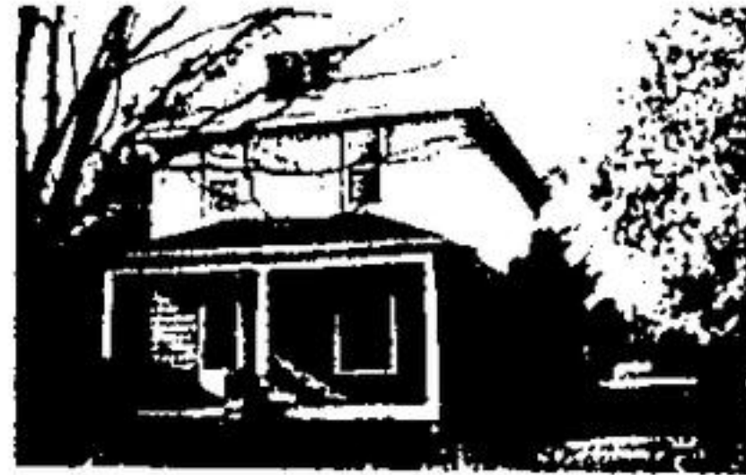
WELL MAINTAINED IN QUIET LOCATION
