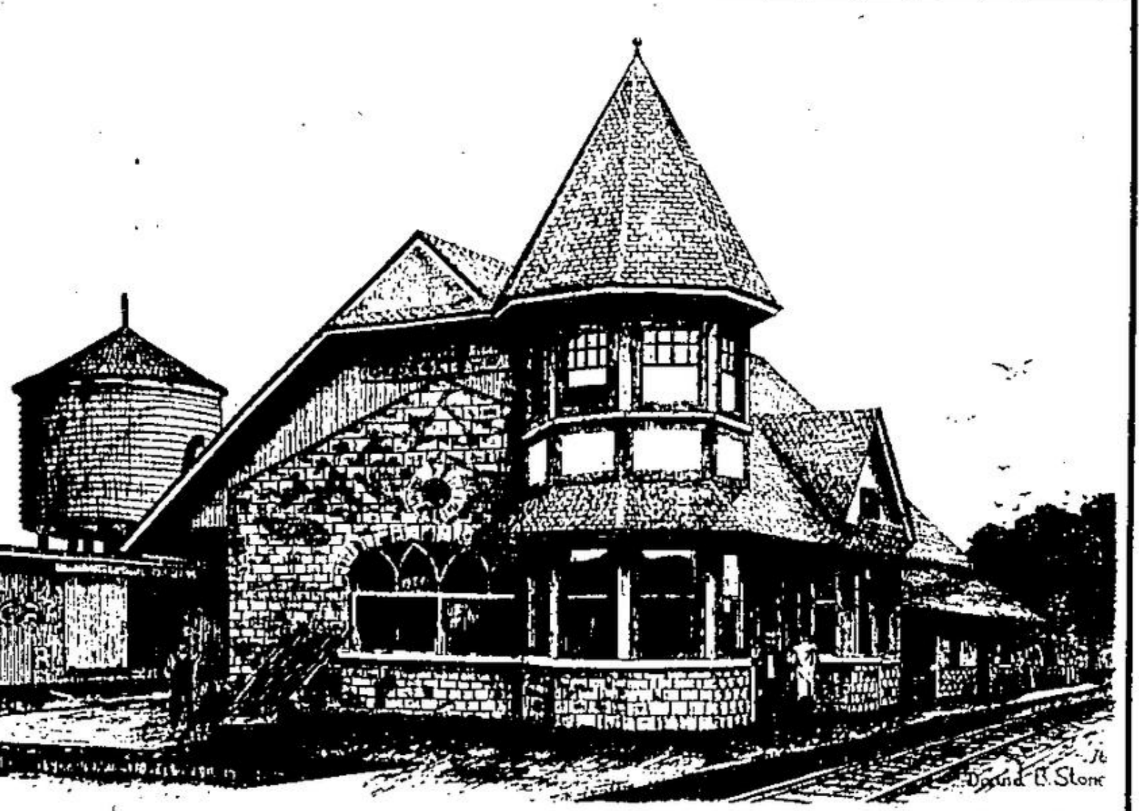
GEORGETOWN TRAIN STATION
