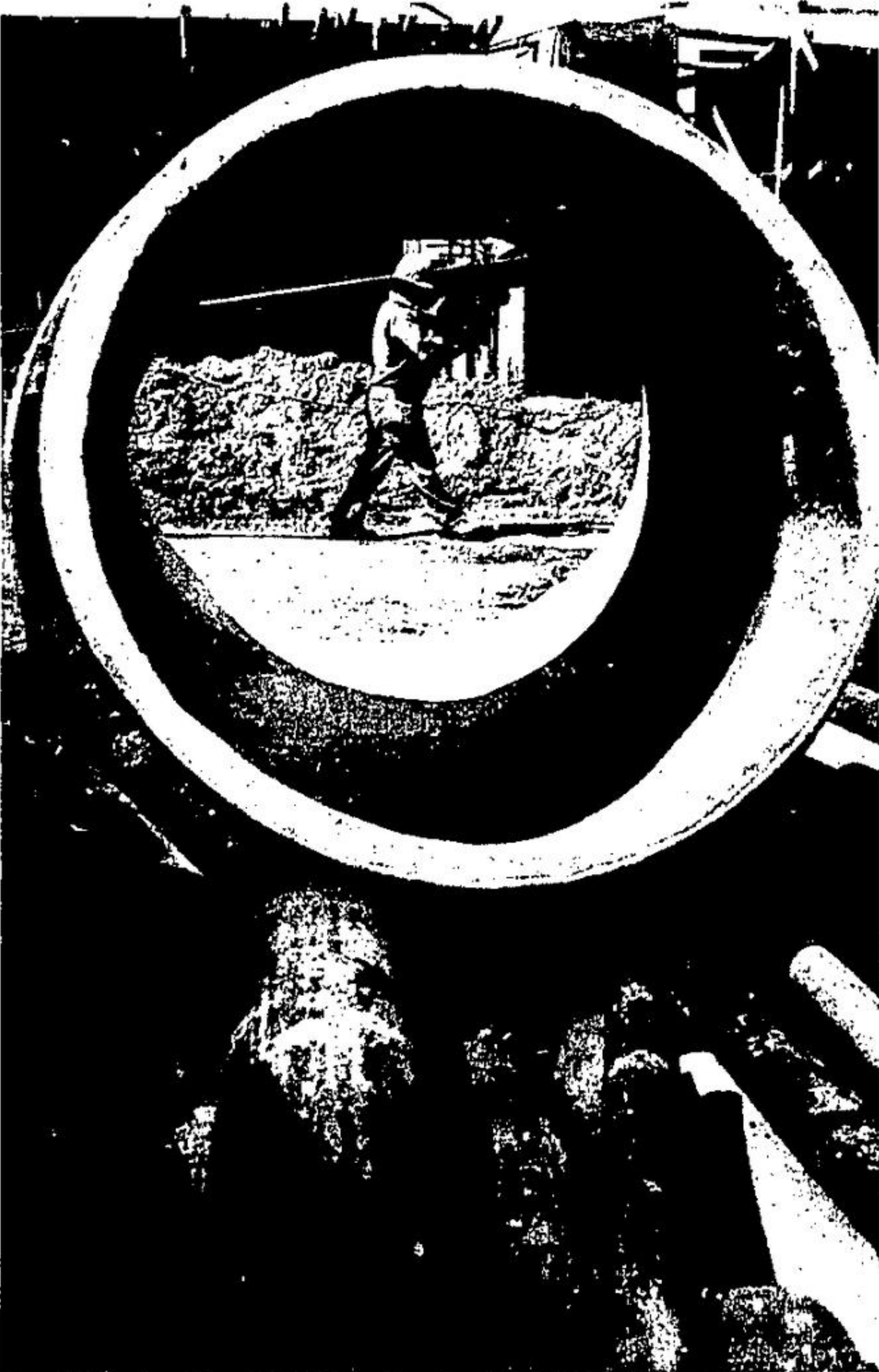
CONSTRUCTION SCENE at the waste disposal site of Mountainview Road near Silver Creek. The expansion to the waste disposal plant is on schedule. It is expected to be completed next spring.
