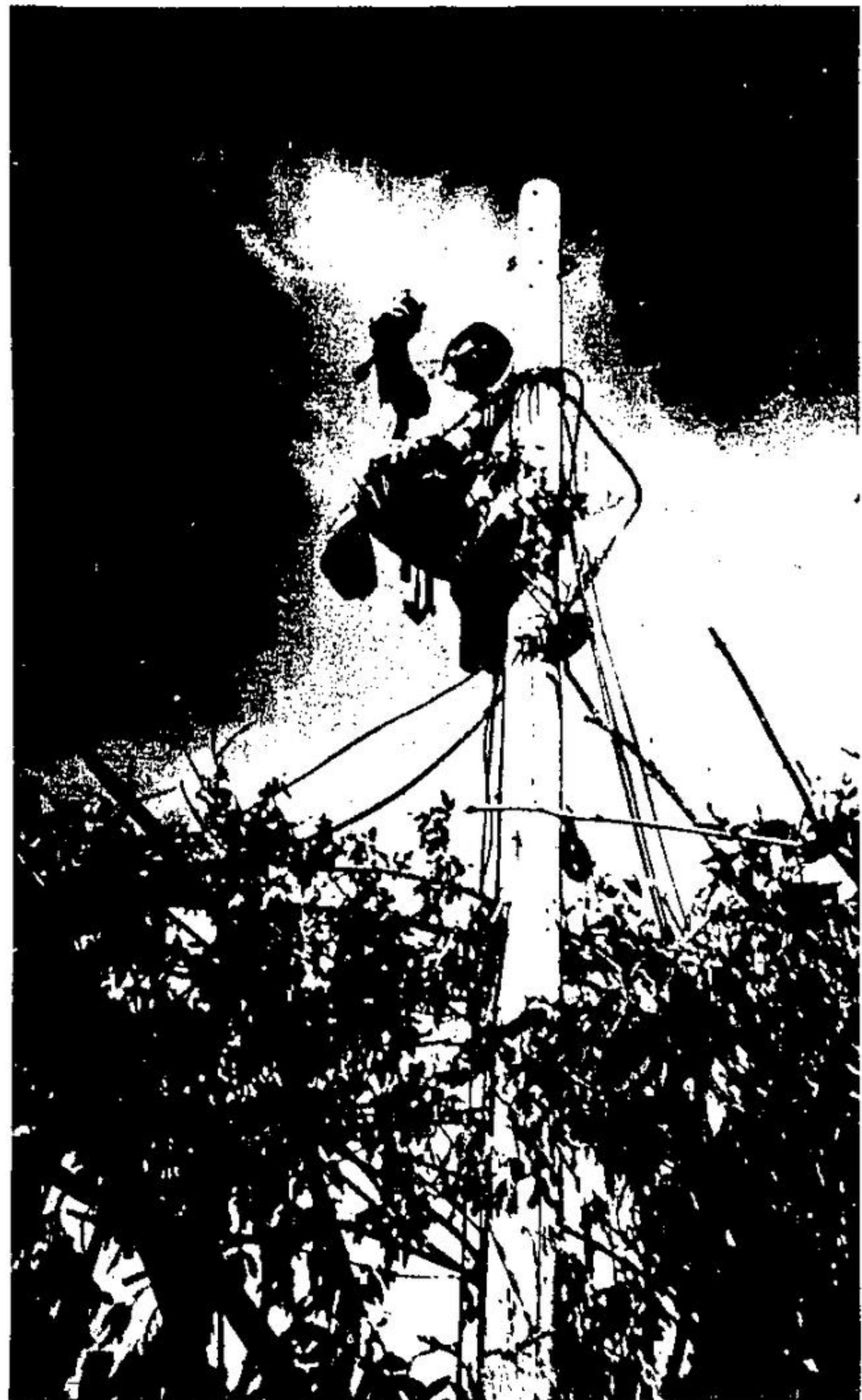
Bell Canada lineman Douglas Anthony at work re-installing telephone lines Sunday morning
