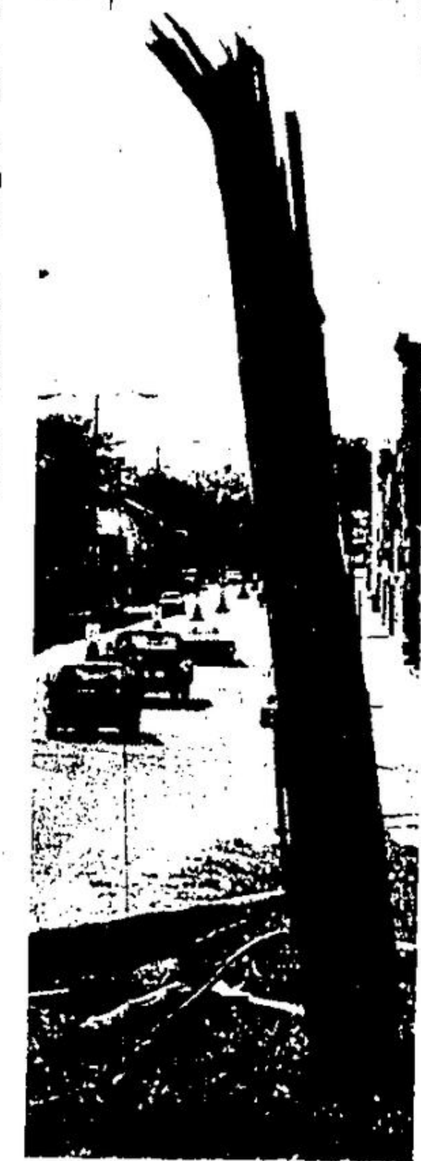
THIS UTILITY POLE was sheared off by the tornado when it struck downtown Georgetown at 3:30 p.m. Saturday.
