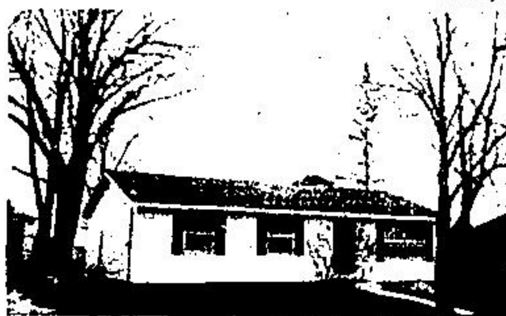
LARGE LOT with trees, new 3 bedroom bungalow located in a characteristic neighborhood, main floor family room with sliding glass doors, fully broadloomed, walkout basement. Ideal for an inlaw suite. Call Flo Matheson.
