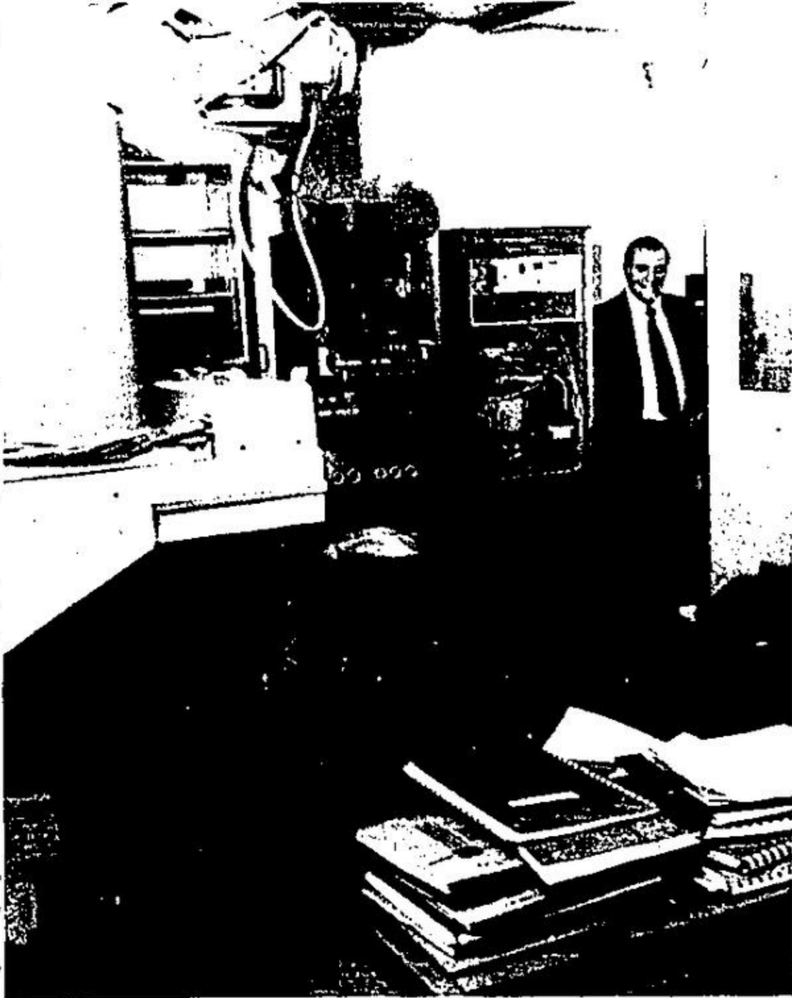
A GROWING HOSPITAL Fred Morris, hospital administrator inspects the construction work being done in the large X-ray room at the hospital.
