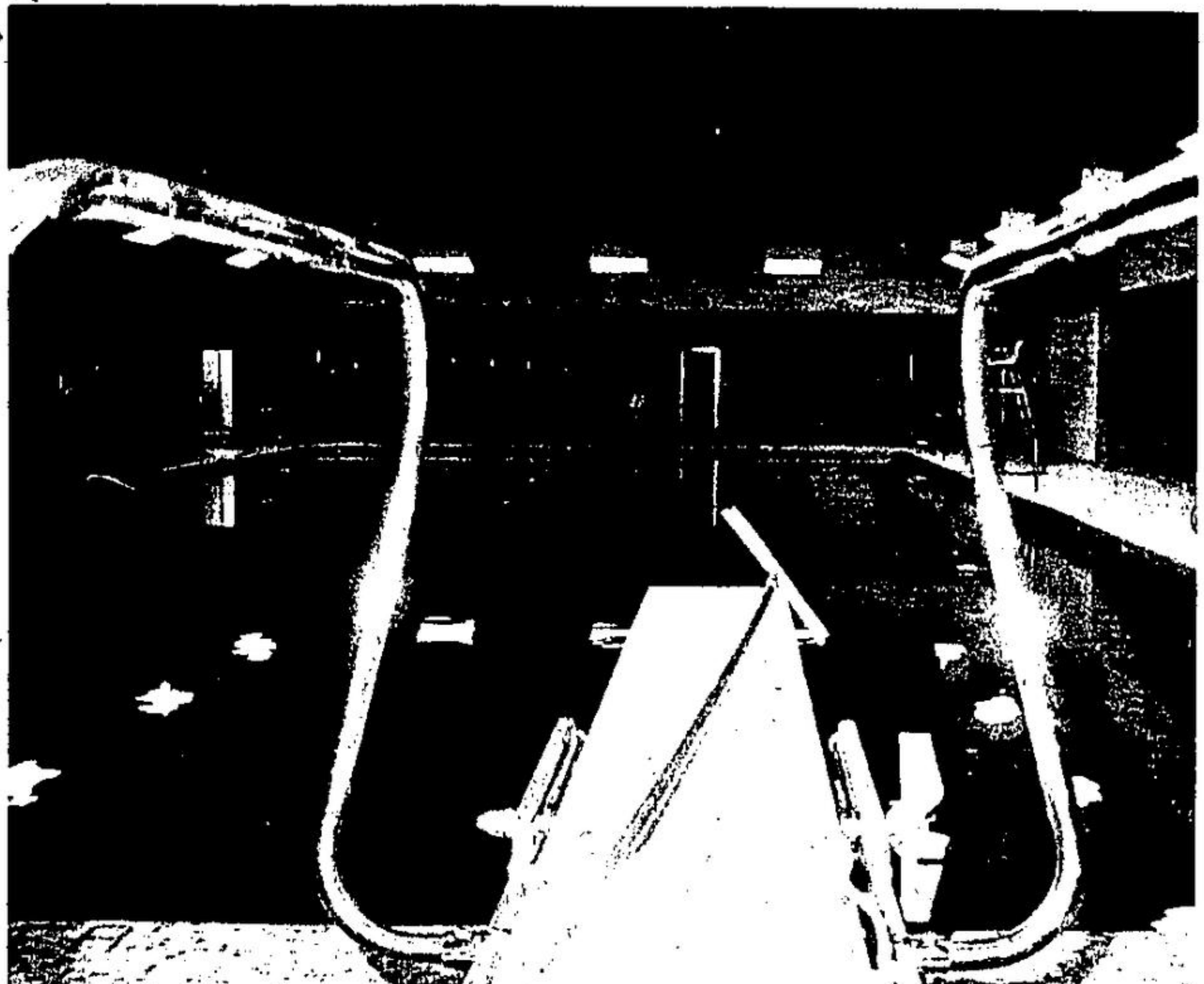
THE ONE METRE diving board provides a panoramic view of the new indoor pool that can hold up to 235 swimmers.
