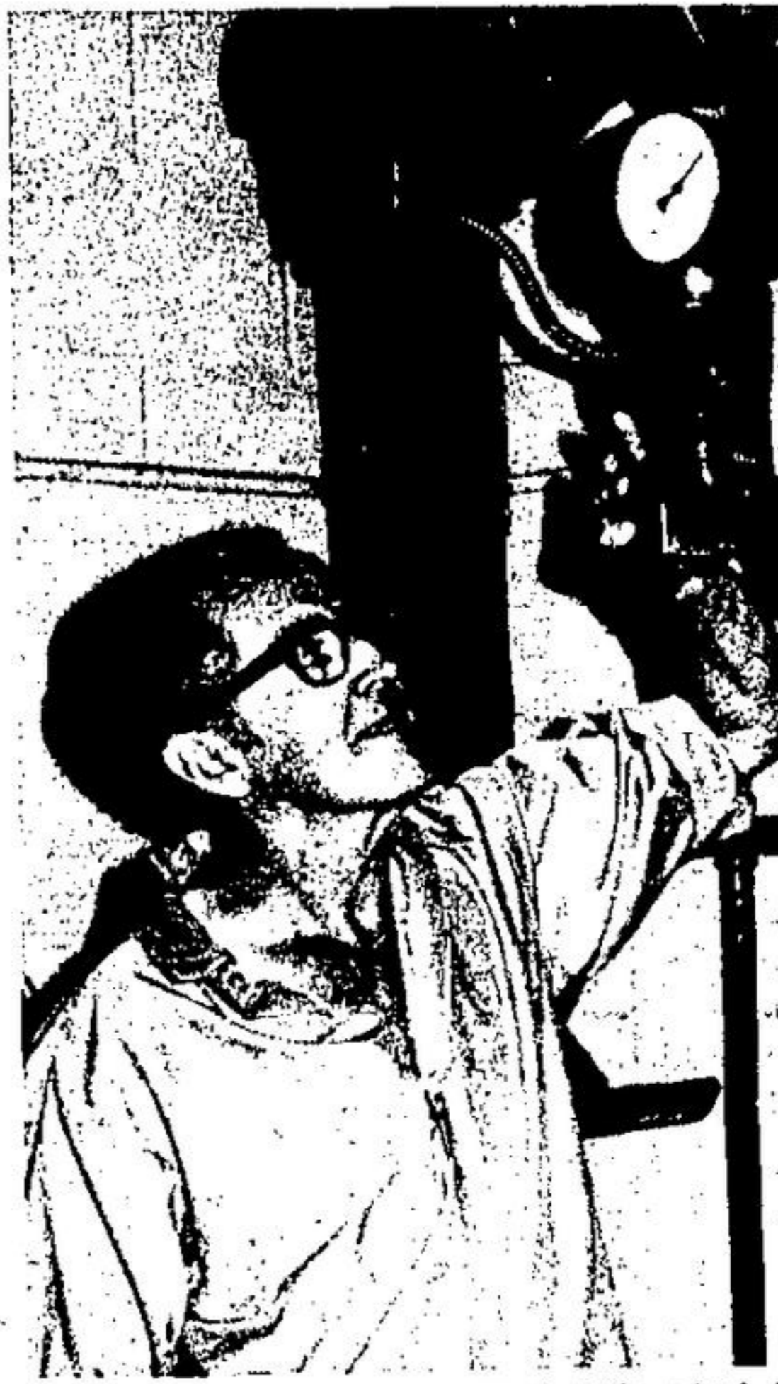
CHARLIE FAYNTER makes a final check of the heating system at George Kennedy Public School in Georgetown before classes resumed at the school this week. School is in 12 months of the year for the regular staff.
