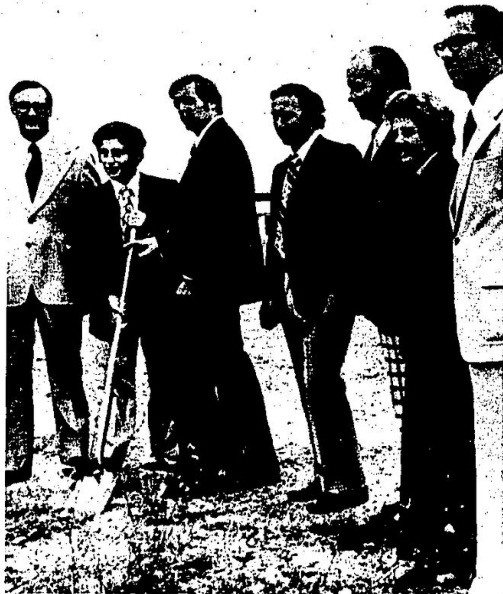
GROUND BREAKING (Herald Photo)
