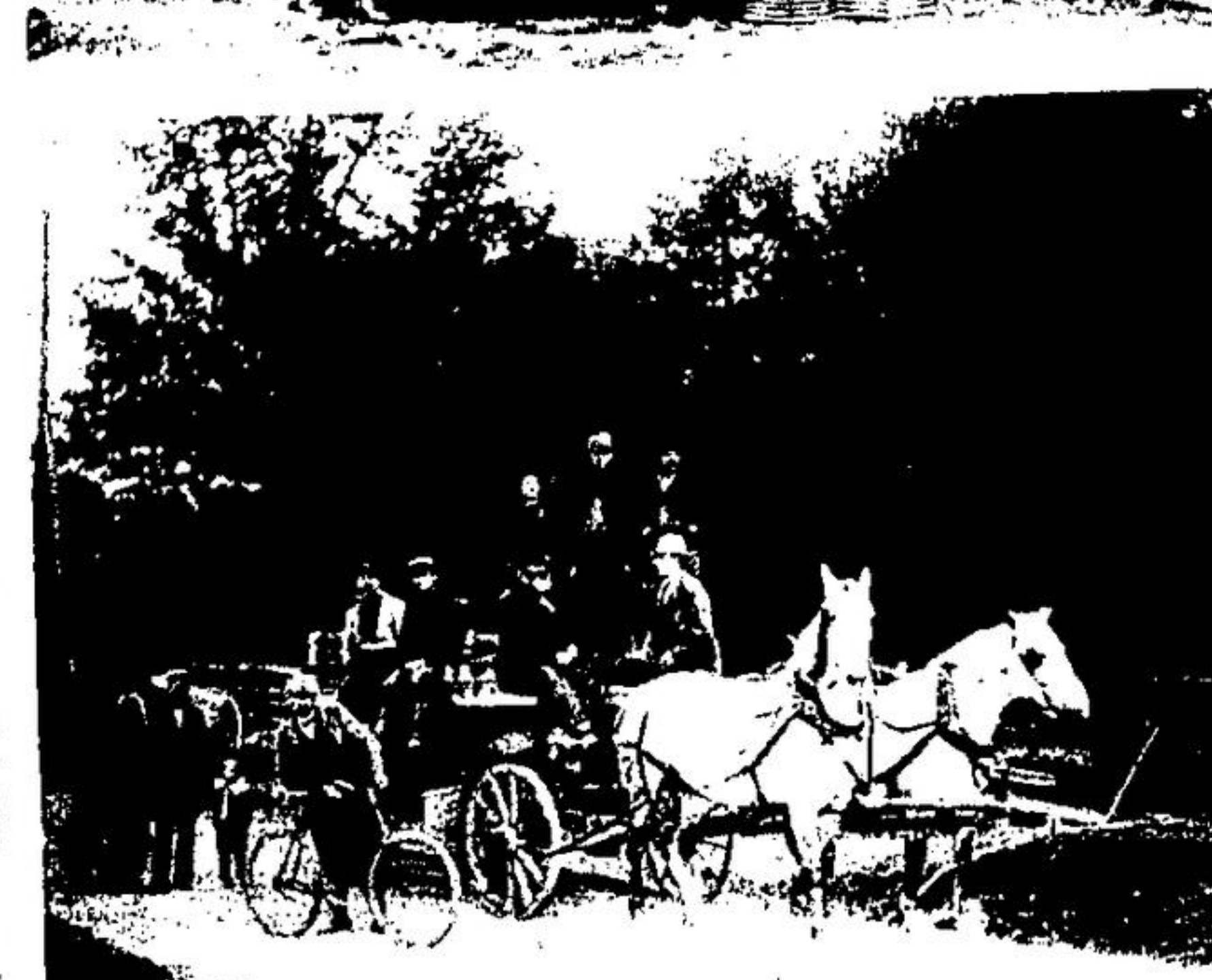
A HYDRO GANG from Toronto putting in a hydro line through Acton. The men would stay at the Station Hotel for four or five weeks until a job was finished. Jean Lasby, at twelve years old would cook breakfast of pork chops, fried potatoes, preserved fruit and toast and coffee for 35 men every morning.
