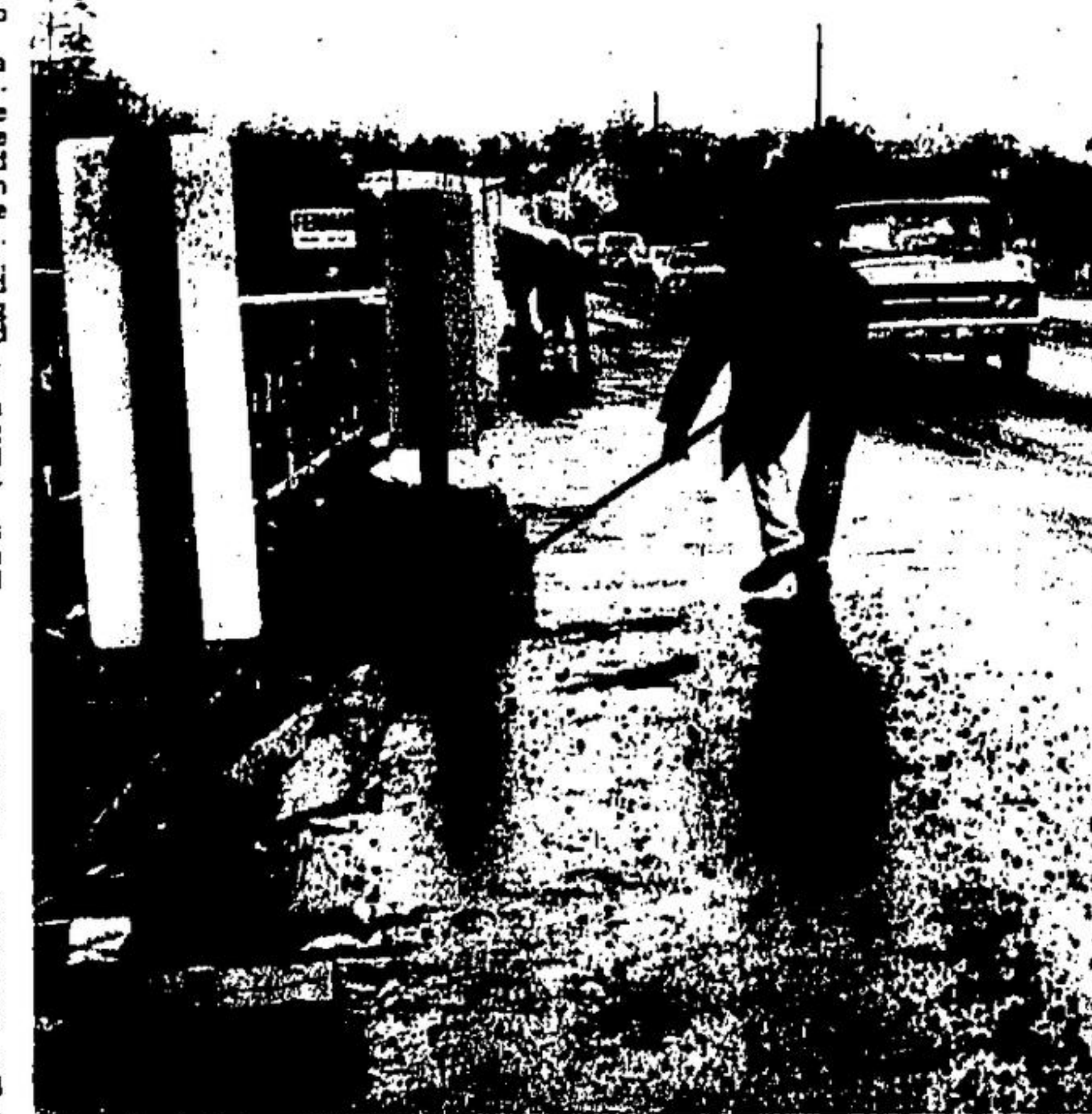
BRIDGE IS SWEEP CLEAN
