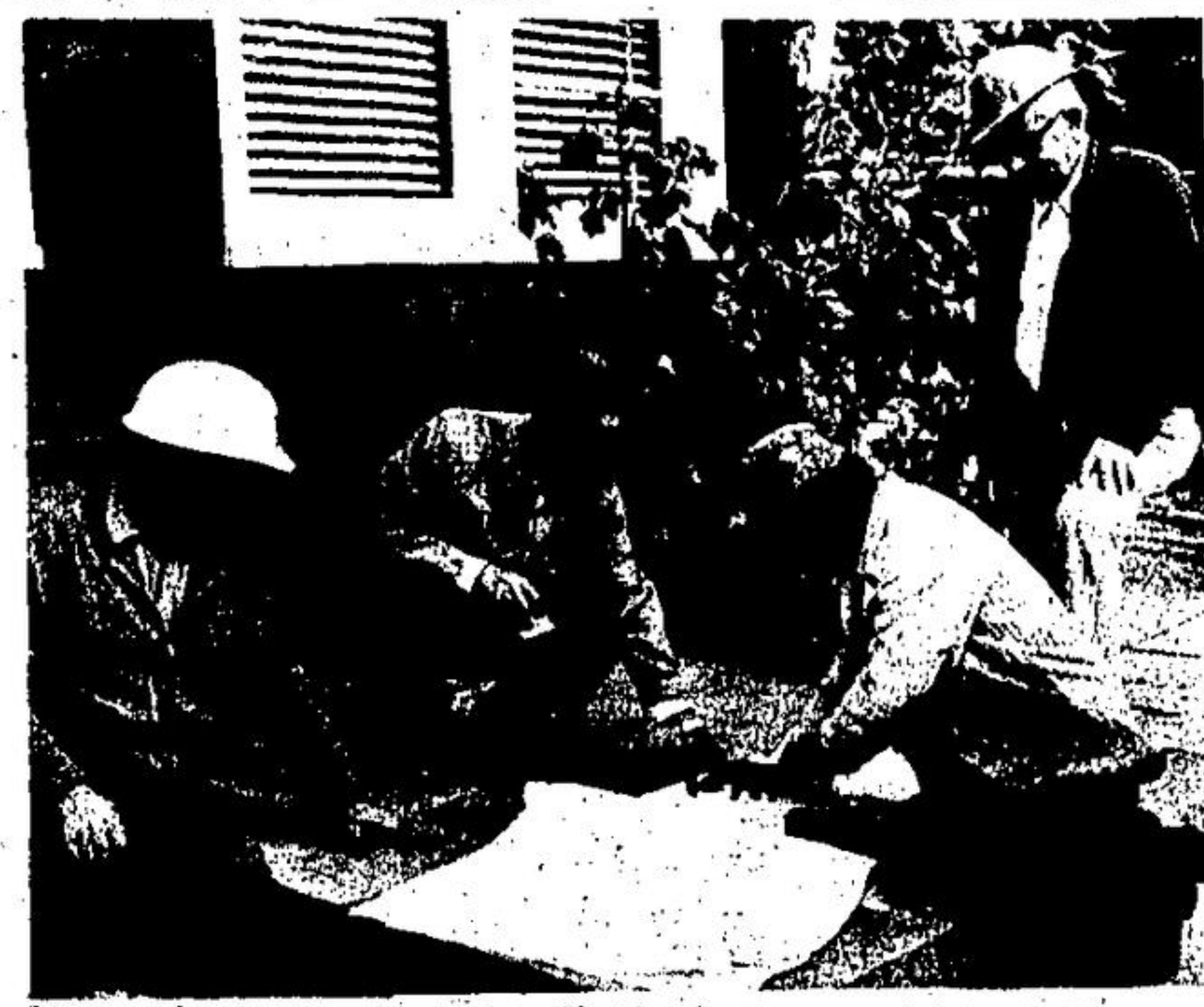
FERMAR PAVING of Rexdale is the contractor for work being carried out at the CN station grounds in Georgetown and the subcontractor is En-San, of Toronto. Checking the plans for storm sewer installations are, from the left, En-San foreman Frank Tericgnl, En-San estimator Hla Shwe, leader operator Joe Stanisci, and Luke McKenna, inspector for the ministry of transportation and communications, Ontario, which operates GO Train service.
