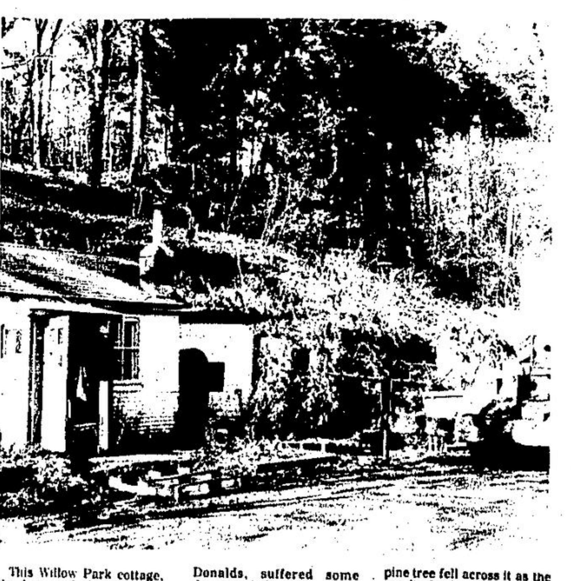
This Willow Park cottage, the home of the Cec Mc Donalds, suffered some damage to the roof when a pine tree fell across it as the result of a landslide.
