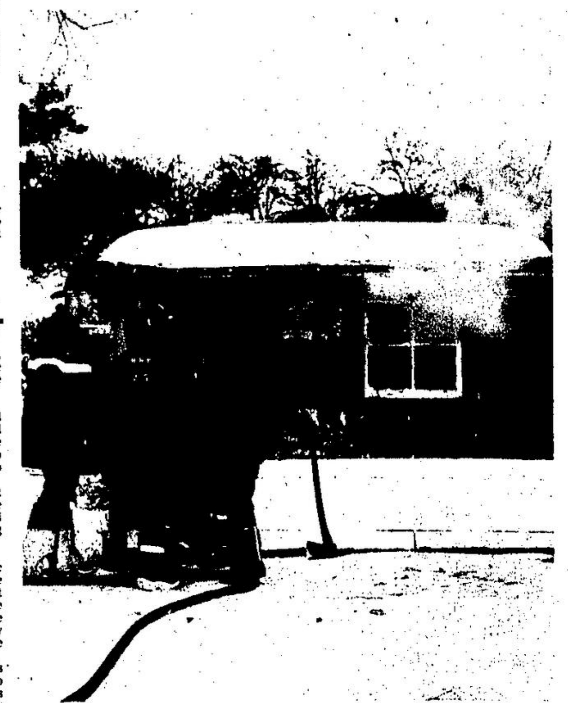
FIRE, FRIDAY, GUTTED TWIN GLEN WILLIAMS SHACK.
