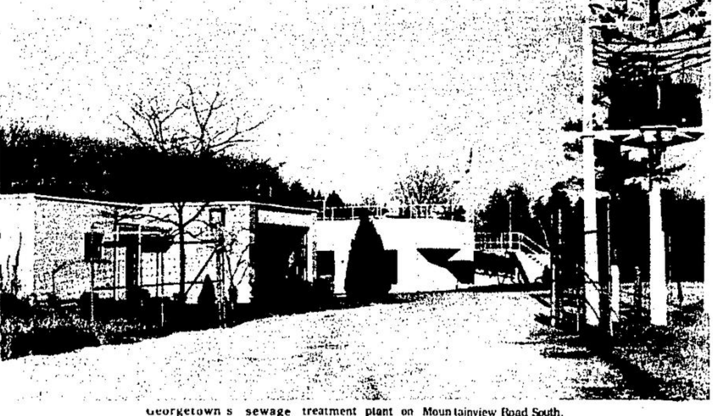
Georgetown's sewage treatment plant on Mountainview Road South.
