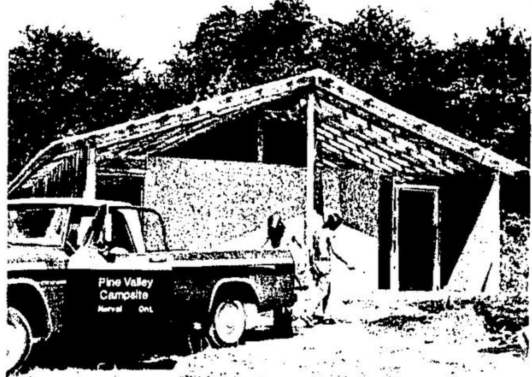
Modern washroom facilities are just about completed.
