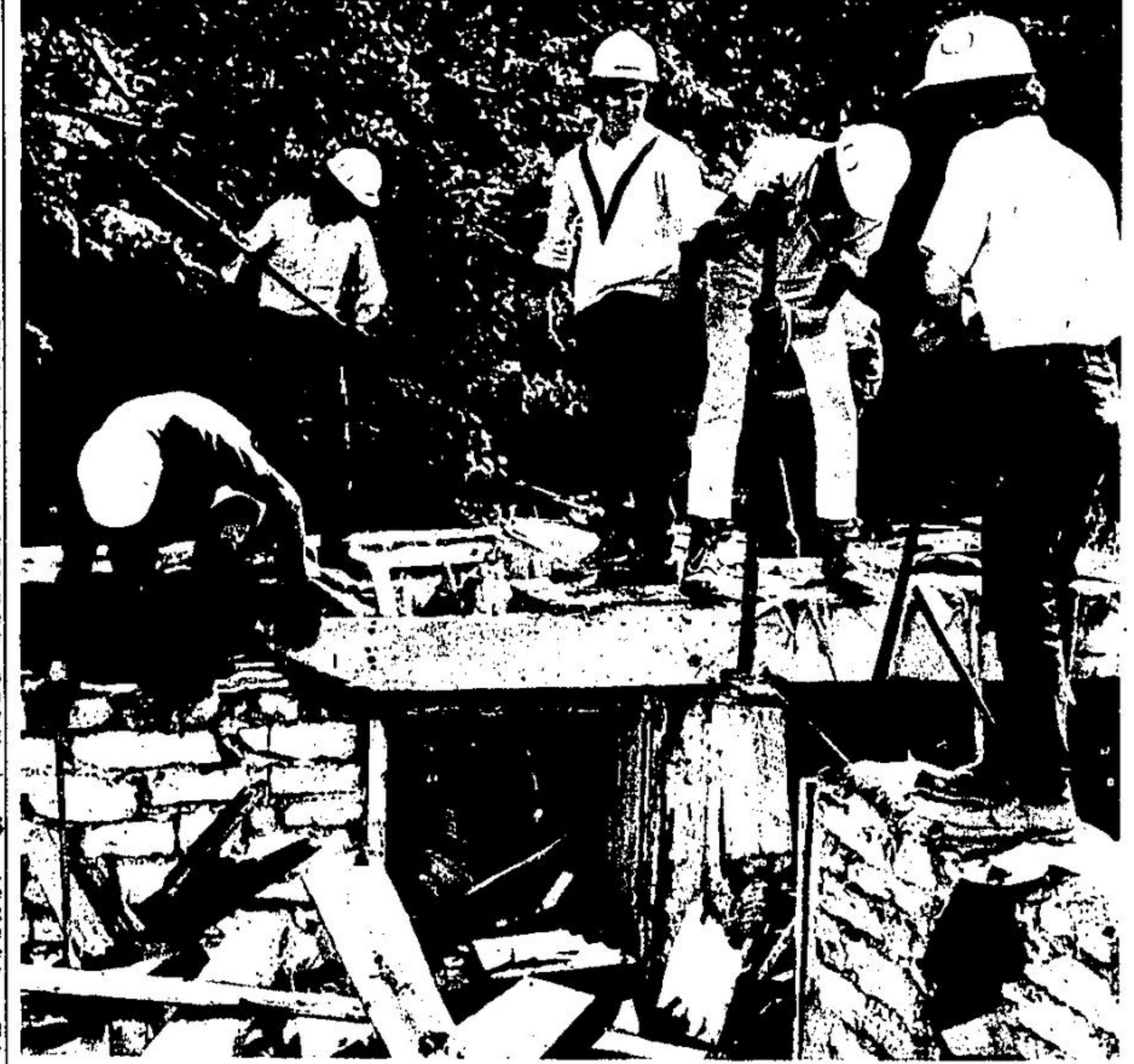
SWEEP students make a demolition crew levelling Limehouse cottage. In the gang are Dave Culliton, John Lavelle, Eric Scratfield, Bruce McKay, Geoff Davidson, Ron Lindsay, Martin Willschick, Alex Love and Rick Currie.
