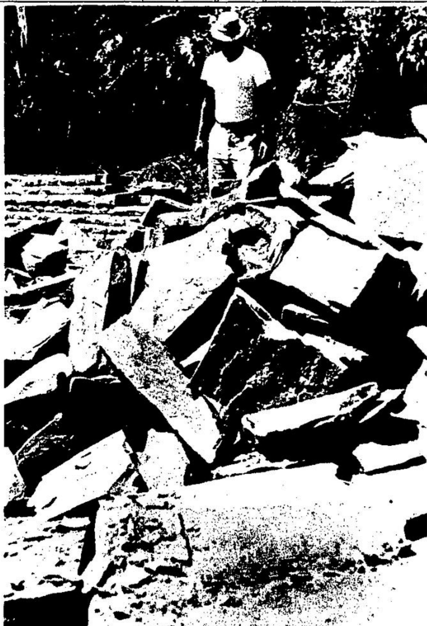
STONE WALL GOING UP
