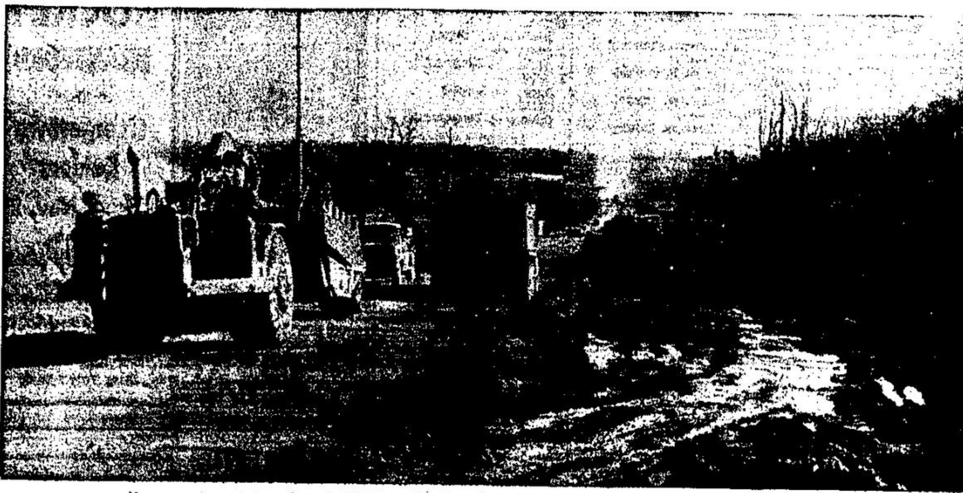
Heavy equipment transplanted 50,000 yards of earth in reconstructing Highway 7 in the Silvercreek area.
