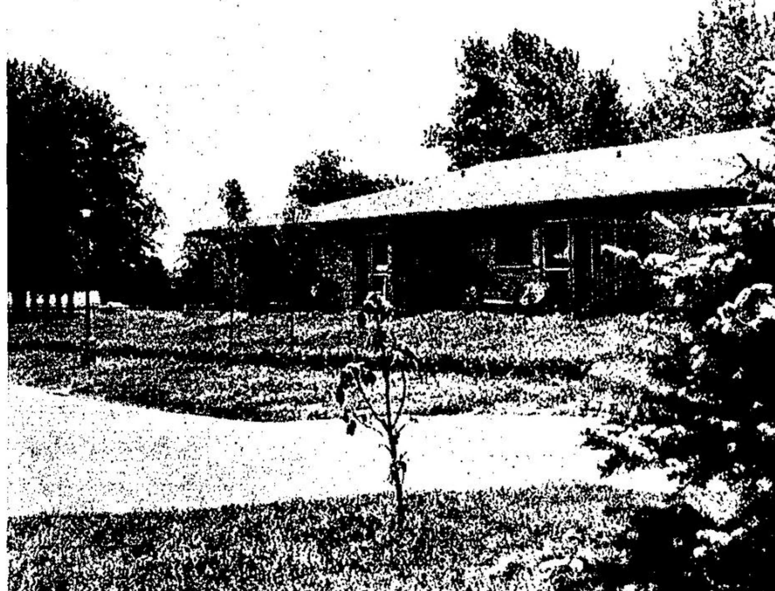
Senior citizens apartments on Hyde Park Drive look more like modern motel.
