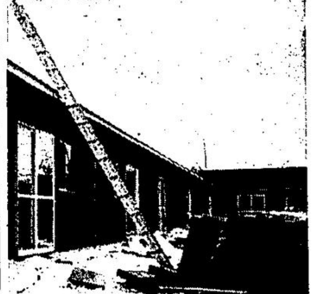
The Kinsmen Senior Citizens' Apartment project on Hyde Park Drive between the hospital and Georgetown park.
