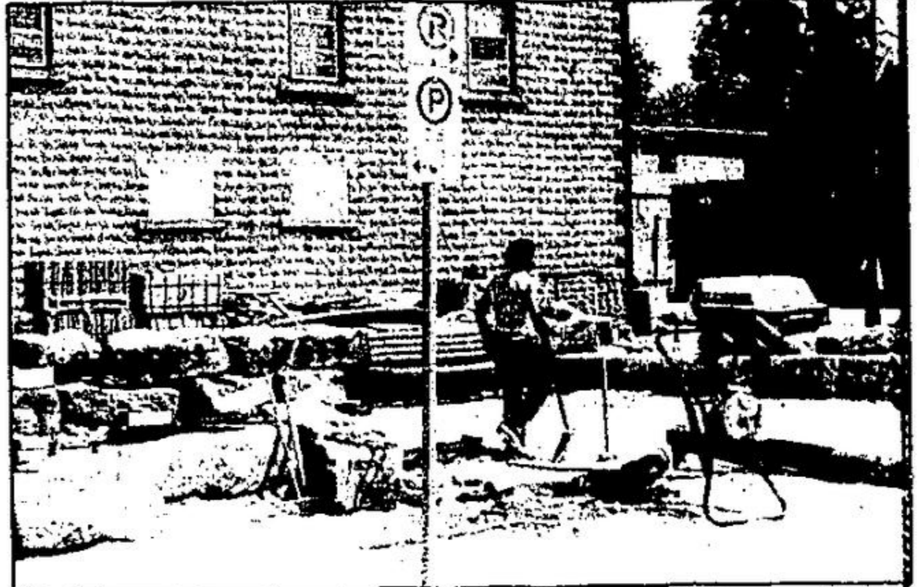
The parkette being constructed on the corner of Mill and Main Streets is almost completed as work crews finish off road and sewer work and put massive limestone blocks in place. An inspector from the Town, who was on the scene, said work should be completed by this weekend.
