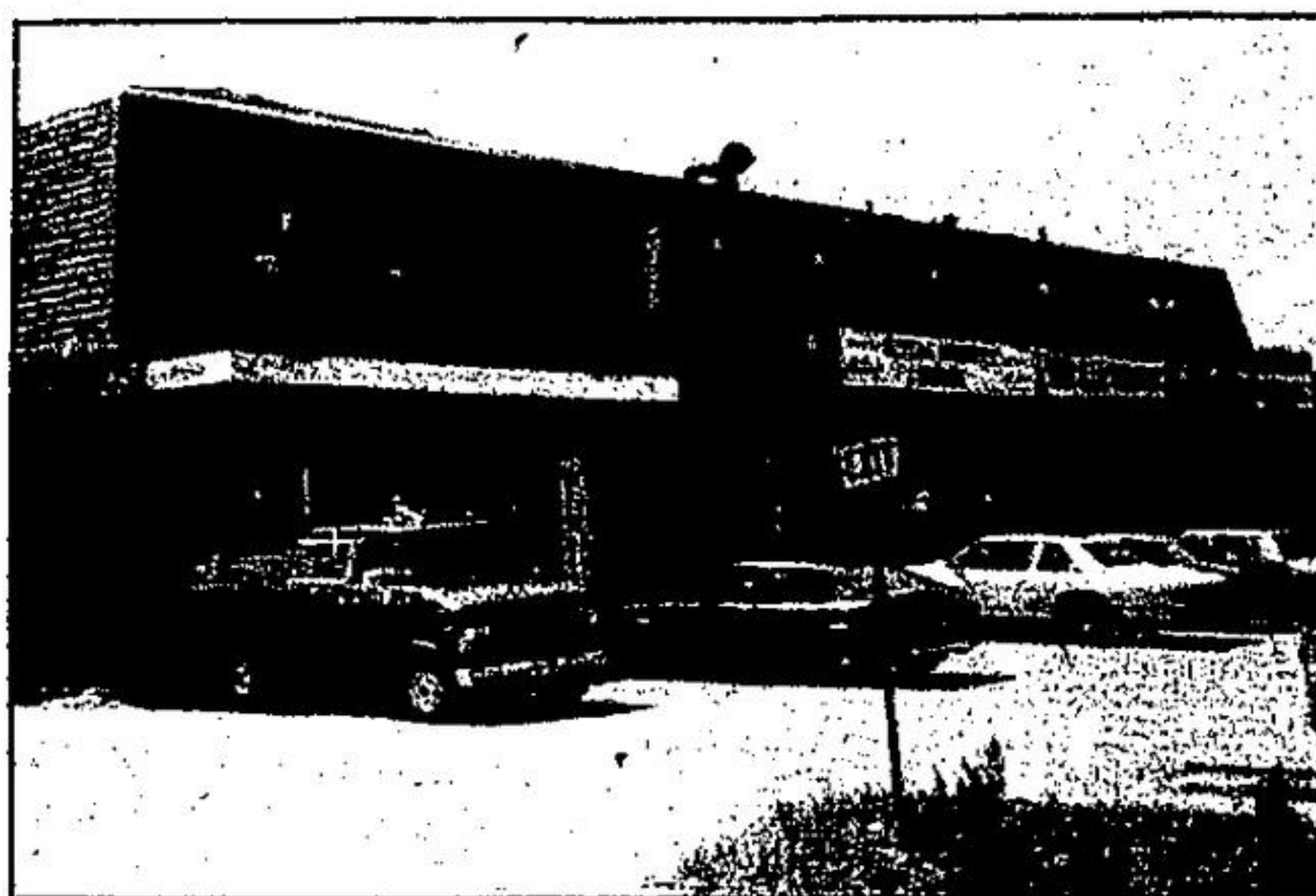
The addition to the Glenlea plaza is almost complete as finishing touches and windows are put into place. The addition has been under construction since April.
