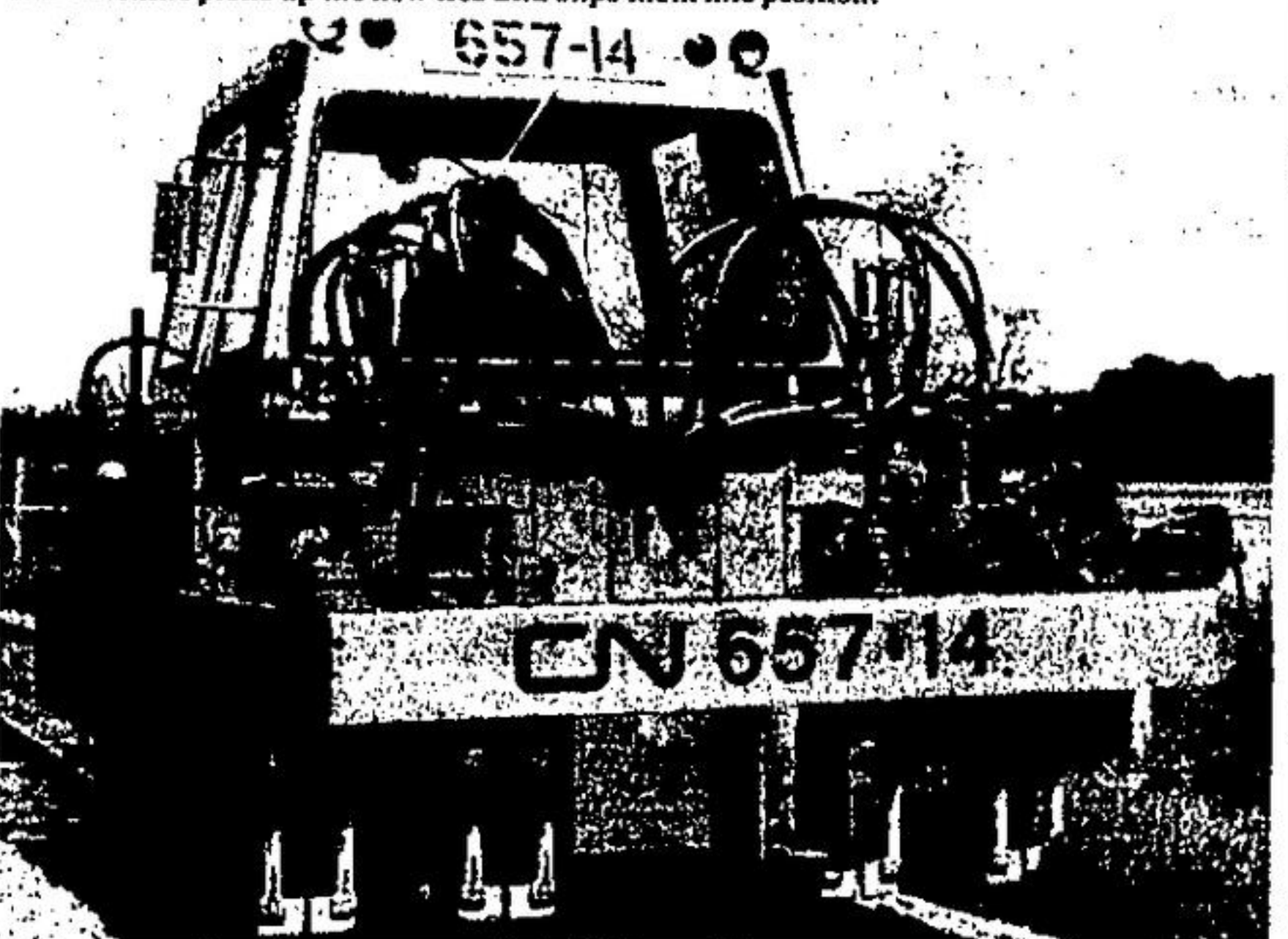
The final step is the spiker which nails the tracks, plates and ties together. Crews on the scene remarked that nearly 600 ties can be replaced each day despite the frequent stops to allow trains through the area. Ivan Hillborn, a CN Engineer on the site, said the work should be completed by the end of July.
