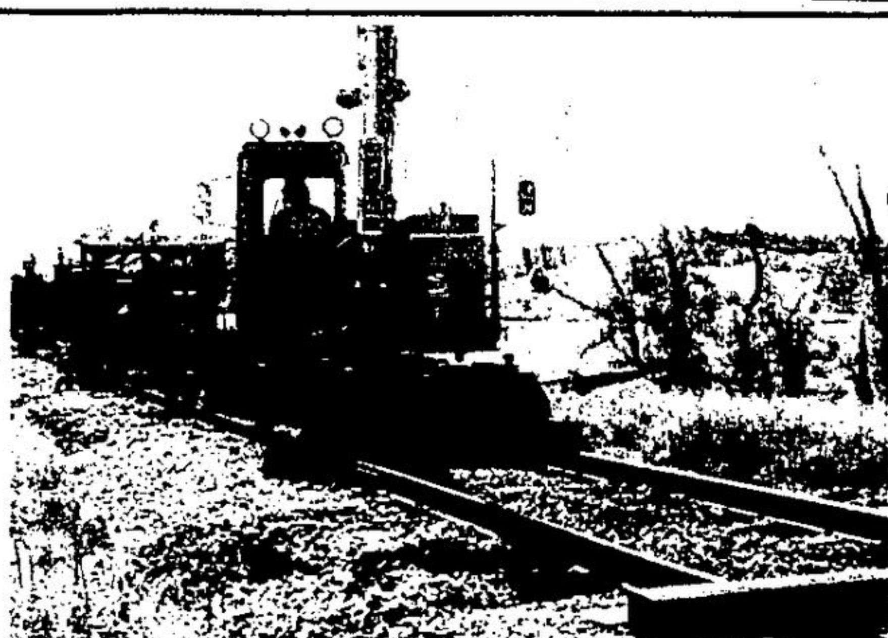
A crane then deposits the new ties on the tracks where they will soon be picked up by another machine.
