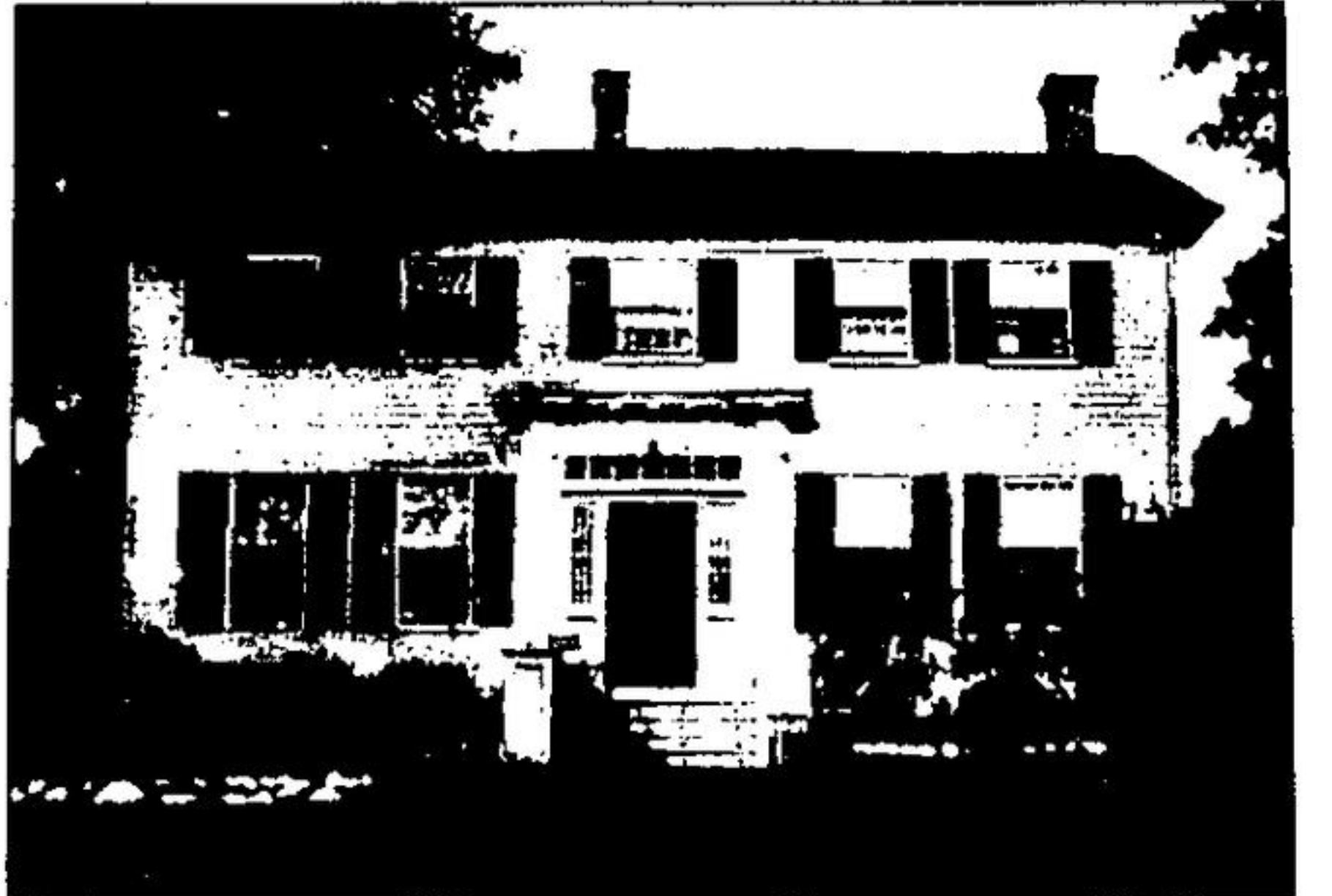
Craiglea, the Stewart home in the Scotch Block, was the first home in the Block made of materials other than logs. It was built in 1832 and there the Esquering rebel, John Stewart, was raised. The home still stands in the Scotch Block.
