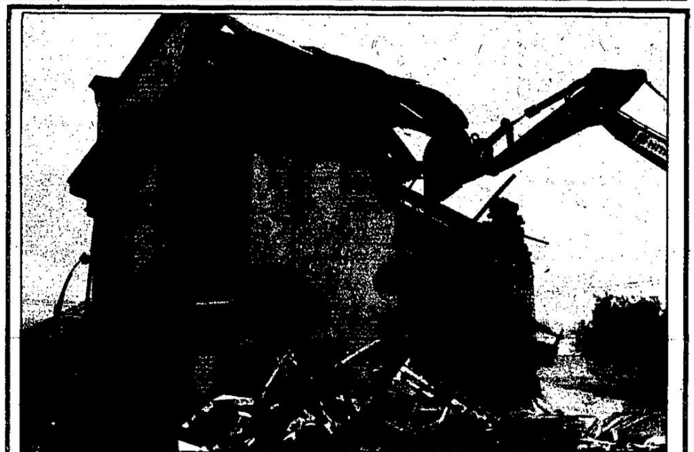
And the walls of Jericho came tumbling down. Well, it may not have been Jericho, but the walls of Acton Pharmacy sure did come tumbling down on Monday. The building was torn down to make way for a spanking new structure. Crowds gathered downtown to watch the demolition as "Red" Lind-
