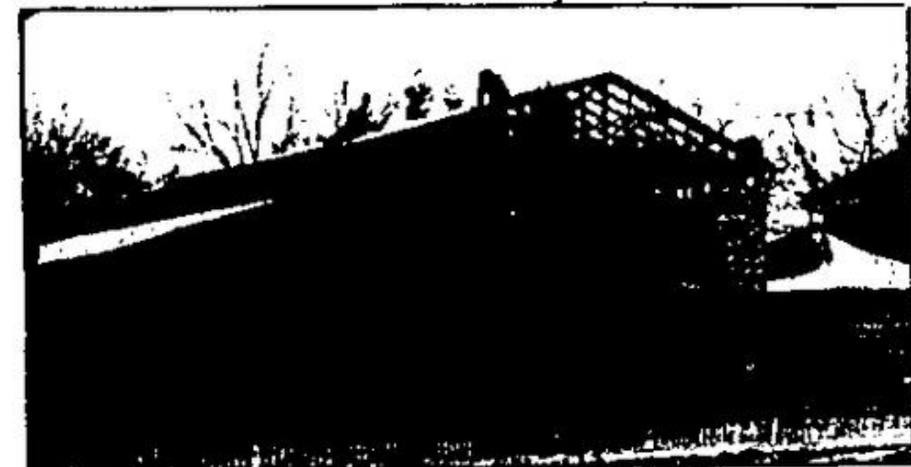
The new Salvation Army Citadel is really taking shape with the roof added this week.
