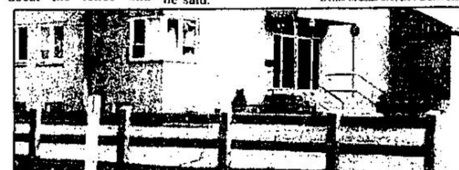
Town workers put up this new fence at Prospect Park last month.
