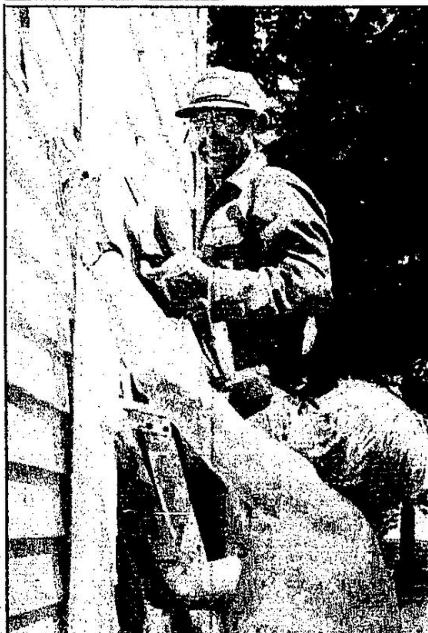
The Churchill Community Church received a new look this past summer as the 144-year-old original tongue-and-groove wood siding was covered with vinyl siding. Here volunteers Jack Denny and Tony Strohov help put on the new siding. —See Page B8.
