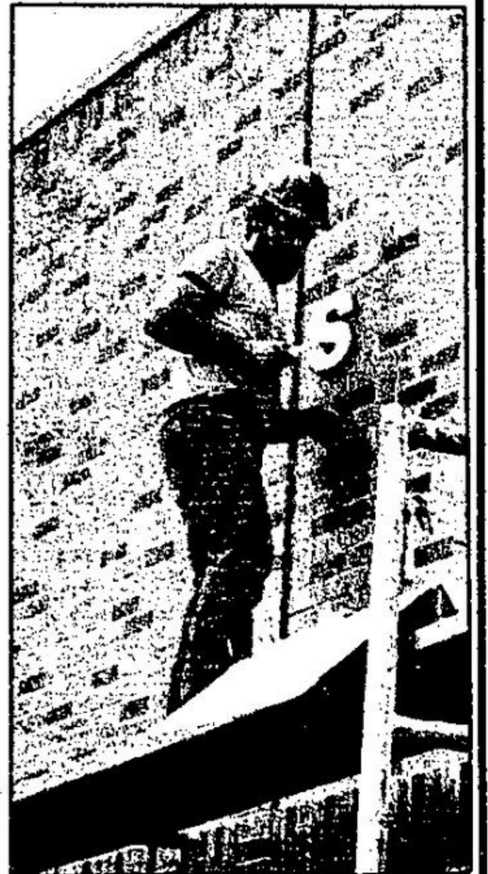
A workman drills holes through the pattern for the St. Joseph's School name which went on the building Thursday.
