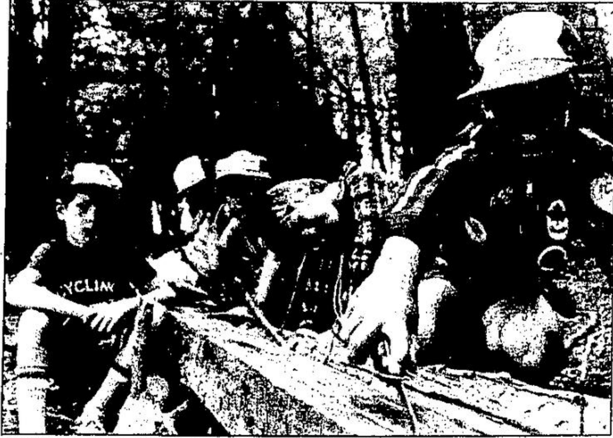
David Hoe works on a bridge while David Chapman, 9, Ben Bailey, Jeff Willis, 8, and Michael Duncan, 7, look on during a camp-over at Blue Springs. The boys decided to build a bridge over some crevices in the bush because girls at the camp had been tripping on it.
