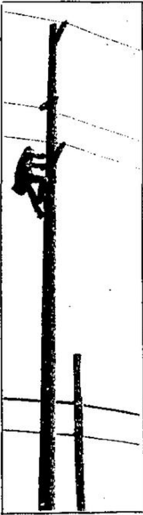
A hydro worker checks an insulator for damage west of Acton.
