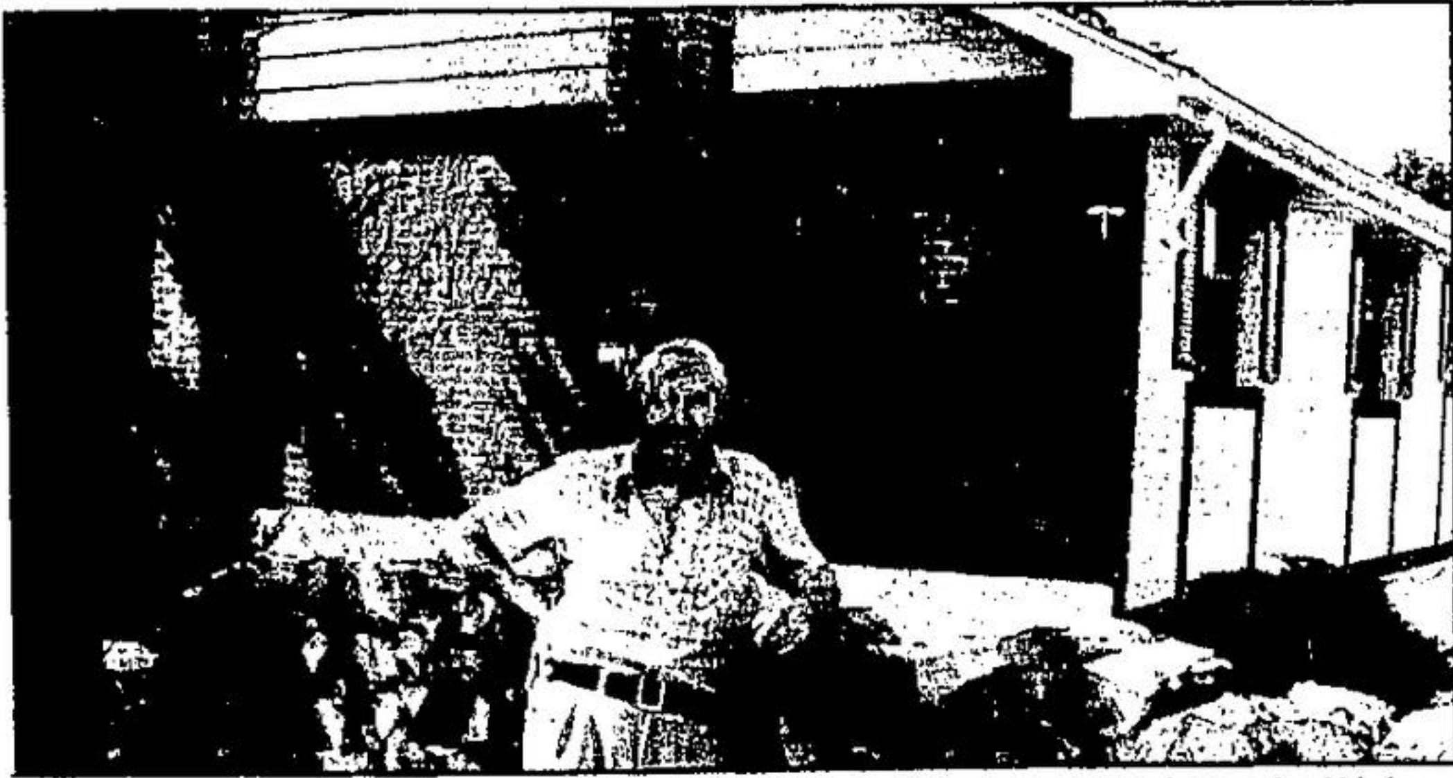
The finished job and what remains to be done. Jack Carpenter stands in front of the brick facade of his home. The facade is to be covered by insulation, just as the rear of the home is to the right.
