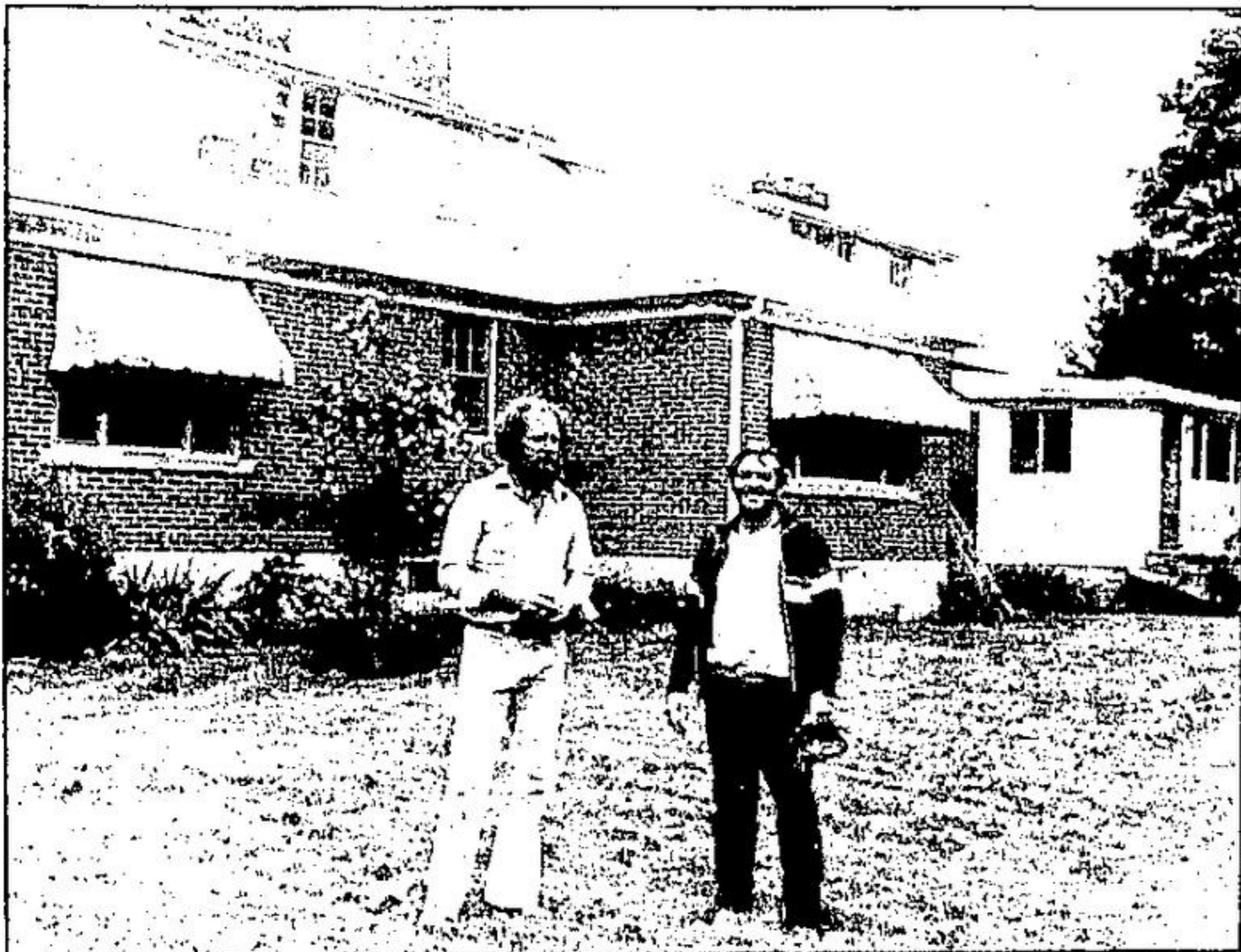
Don Cave, left and Dave Dineen, two members of the executive of Halton Hills Centre, discuss renovations inside and outside the house. A three-car garage is being converted into three bedrooms and a bathroom, and there are plans for building a glass enclosed dining area to the back of the house.
