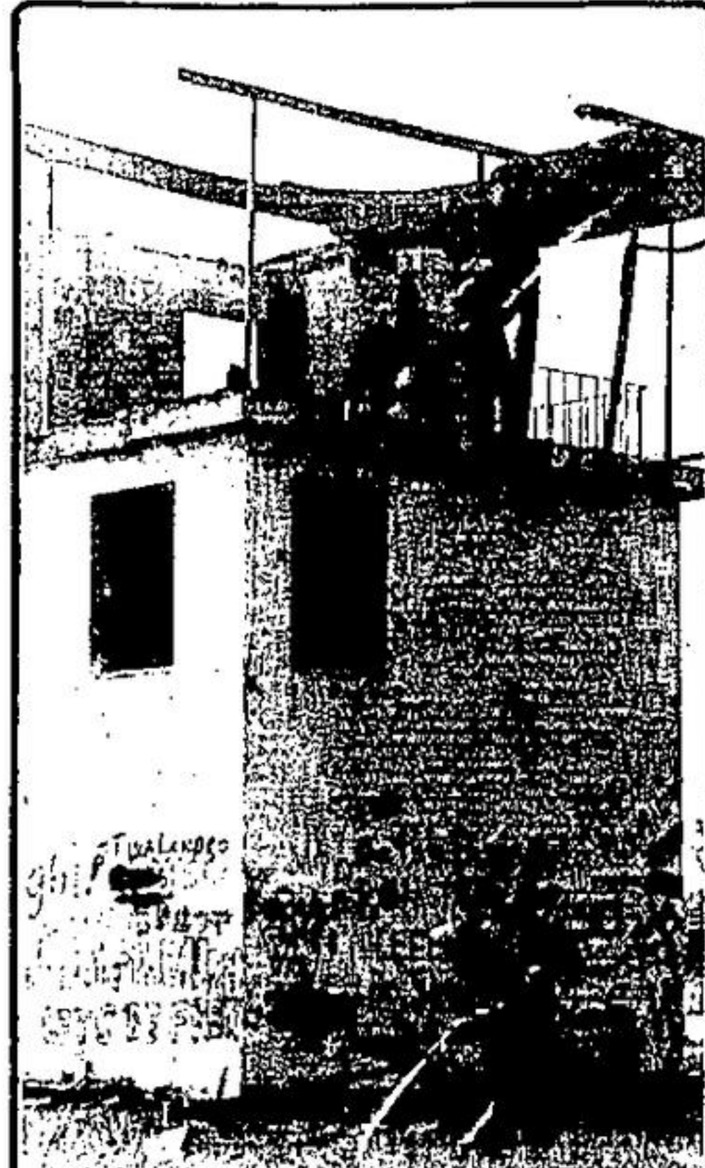
Acton Firefighters were called out three times to battle flames at the control tower on the grounds of the old drag strip last week. Firefighters say the fires were set.
