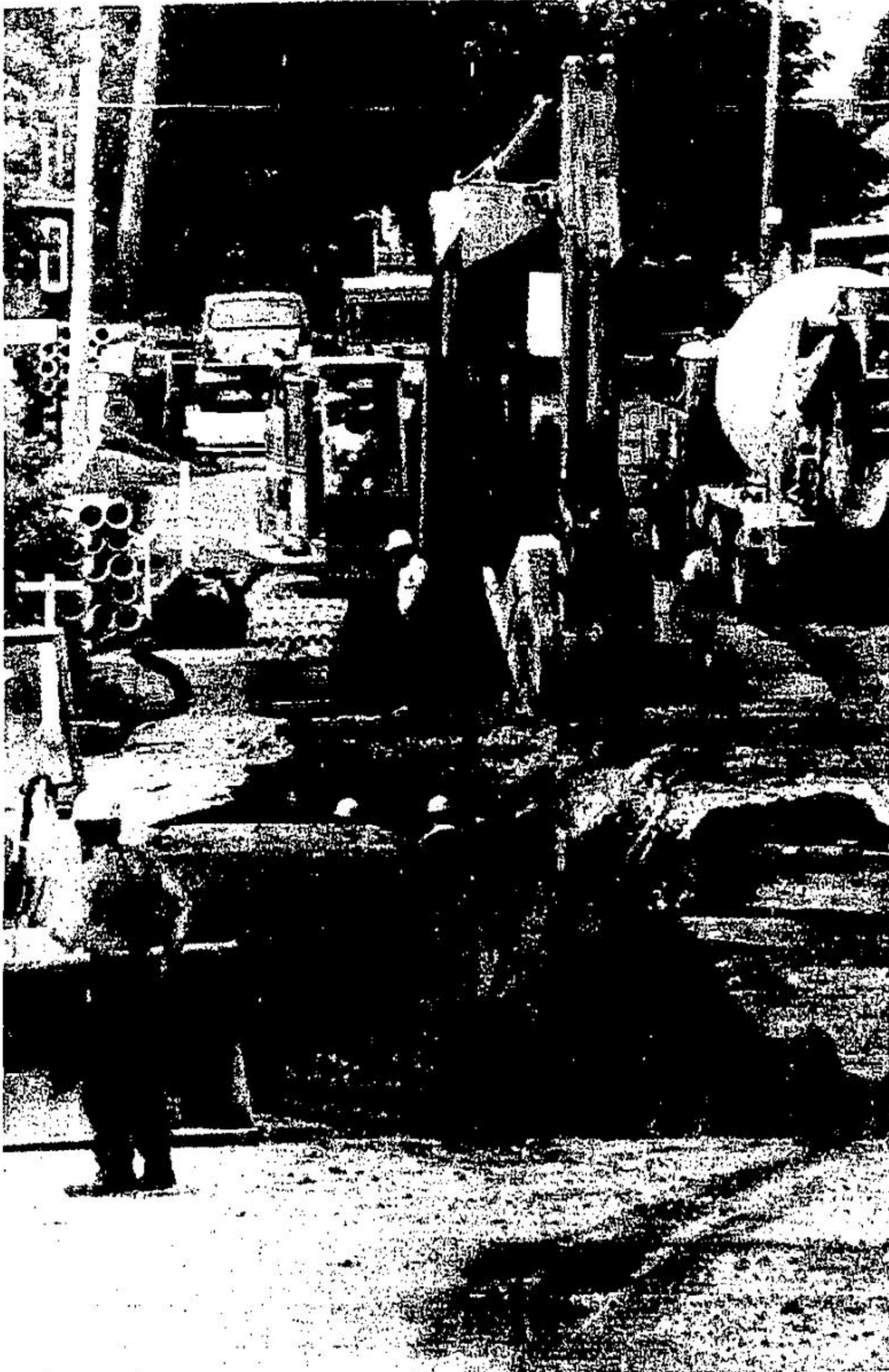
Mill St. W. between Victoria Ave. and Cameron St. is closed off because of the work of sanitary sewer replacement. Lamco Construction, of Markham, has the $1-million contract for that project and some others in town. Halton Region and Halton Hills are sharing the cost of the job. On Monday, work centered on the road between the dam and the flour mill.
