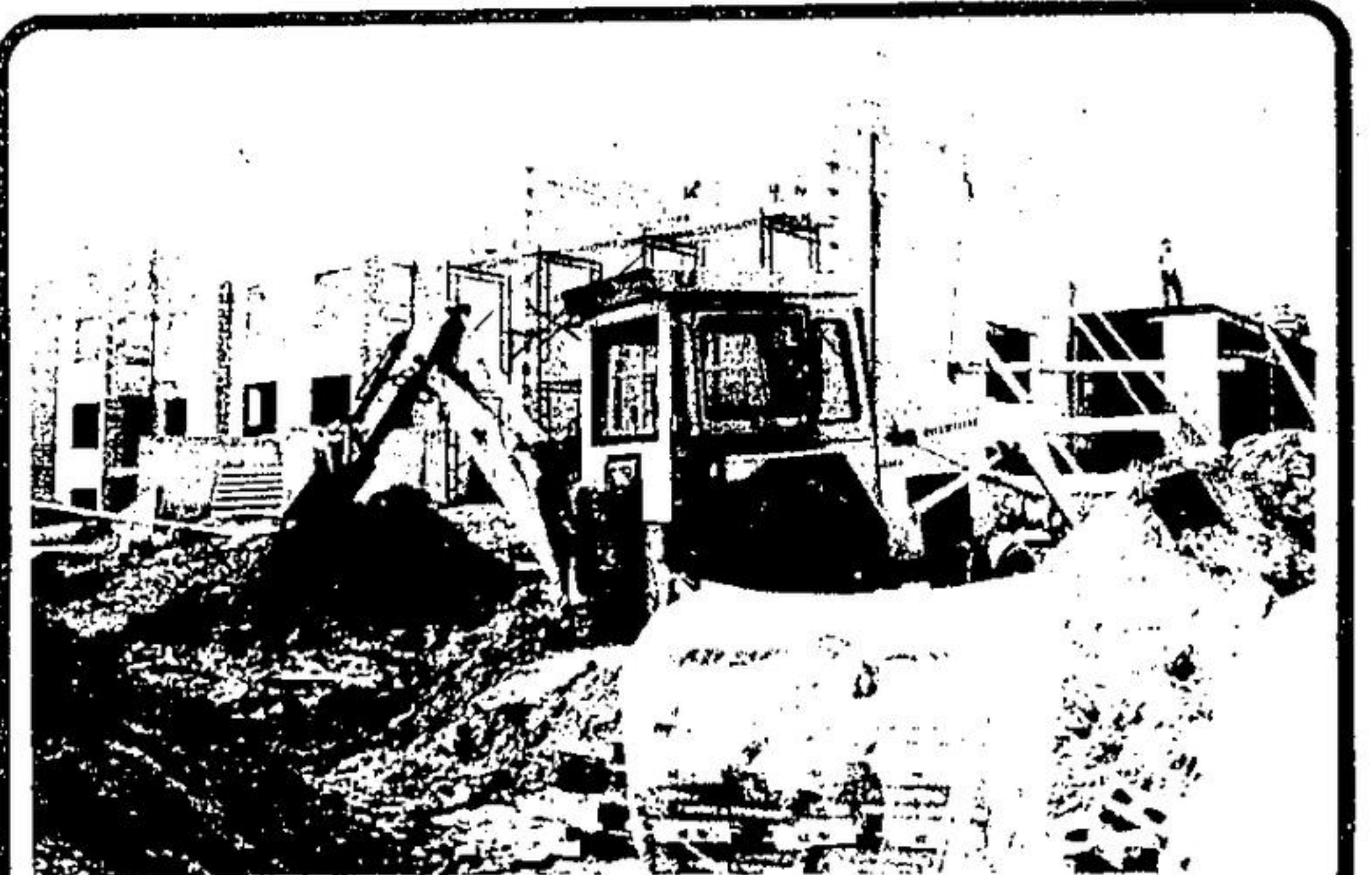
Things are starting to take shape on the north side of Fairy Lake at the senior citizens development contracted by J.P. Dumarche Construction. The building is scheduled for completion in March of 1980.
