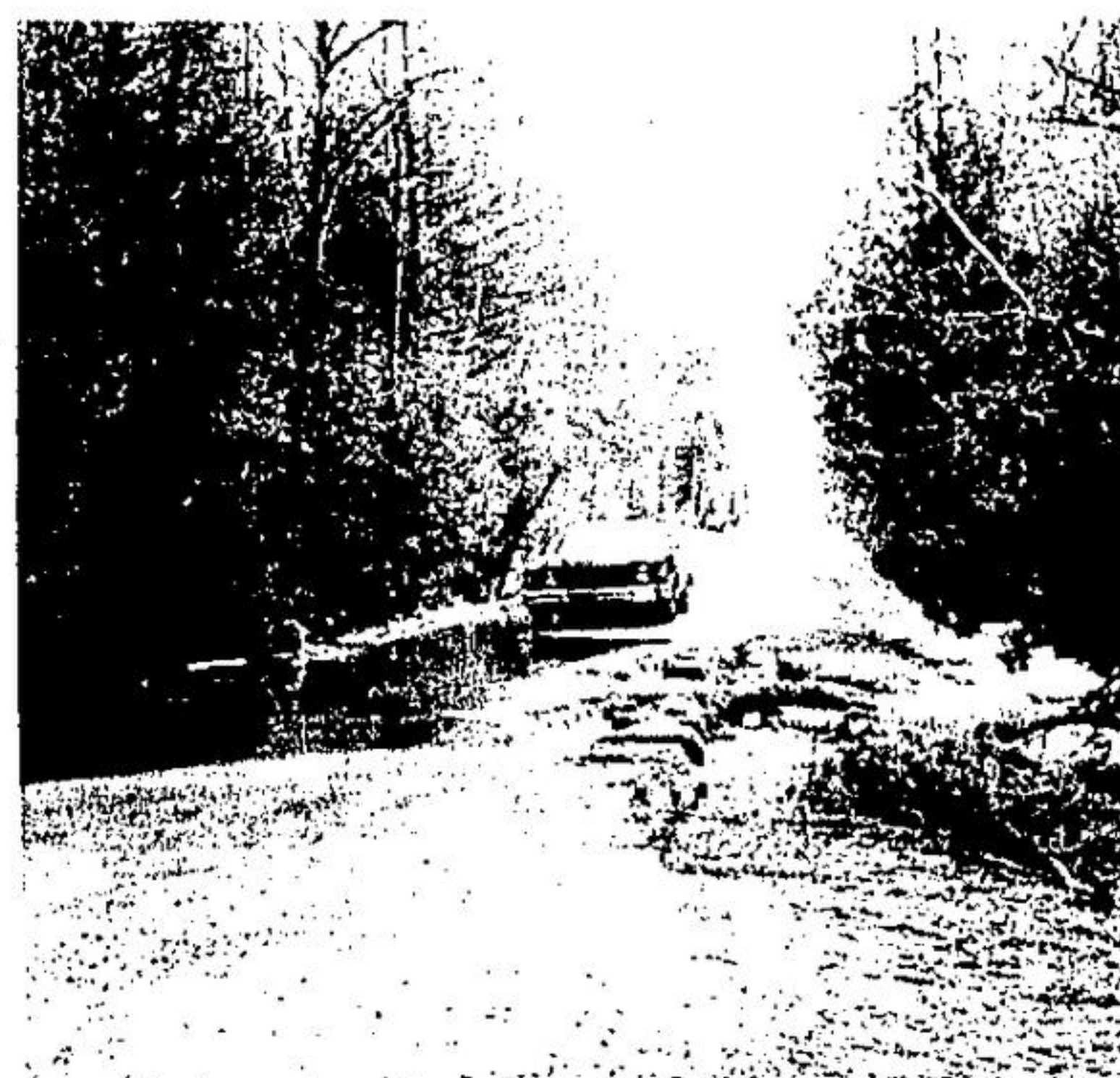
Copious rains last Friday and melting snow inundated some rural roads in the Acton rural area such as this First Line road in Erin township, just north of the Acton Meadows golf club. The surface caved in where a culvert conveys a tributary of the Blue Springs Creek under the road.
