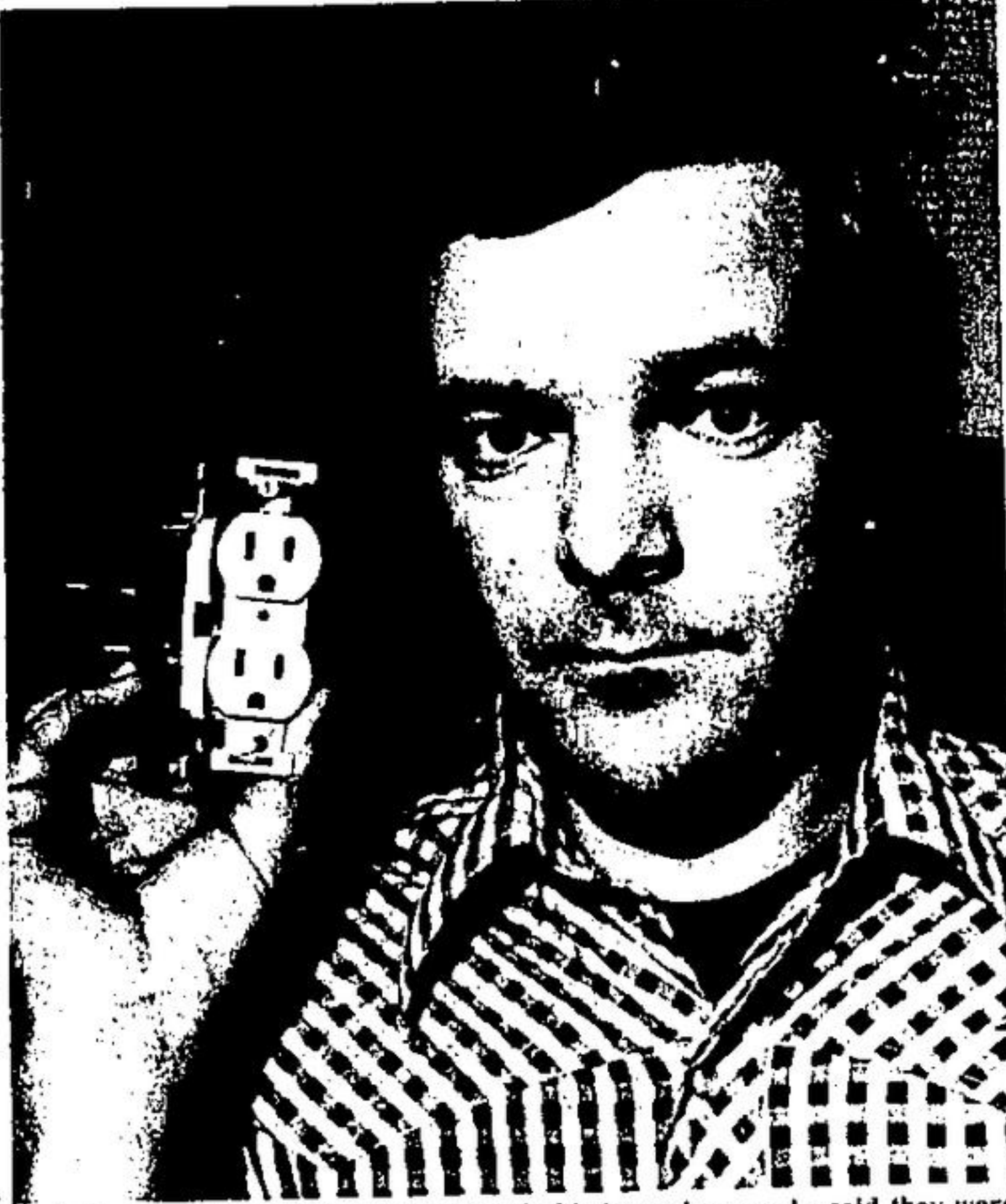
Arch Harkins replaced the wall sockets in his home because he said they were overheating and arcing. The sockets were discolored and much of the wire covering burnt off.
