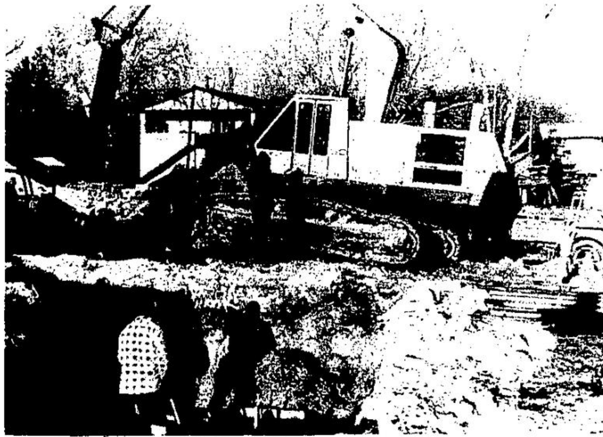
J.P. Ducharme Construction Limited from Zurich, Ontario has begun the foundation construction of the new senior citizens' apartment development on Elizabeth Drive, north of Fairy Lake. At present the work is being completed as weather permits.
