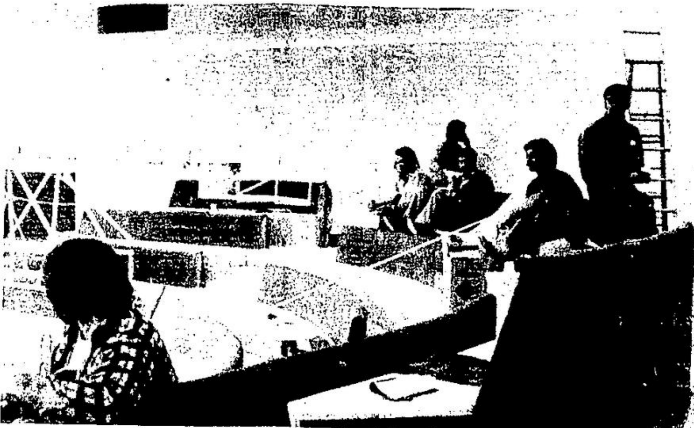
COUNCIL IN THE ROUND is the format the new council chambers of Halton Region is taking in its new building on Brante Rd. just north of the Queen Elizabeth Way. The circular design allows everyone to see everyone else. Workmen take a coffee break during construction.
