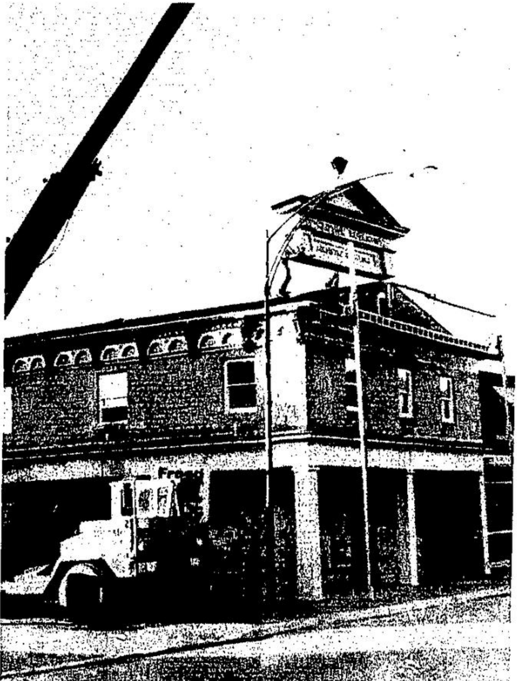
CROWNING GLORY... the original old top of The Old Free Press building was hoisted back into position atop the new building Friday morning. It was securely bolted from the inside by Doug Fread and Peter Schmuki. The building is reconstructed in the style of its 1904 predecessor, with decorative mouldings newly cast from molds of the original old pieces. Block and pillars closely resembles original tinwork.
