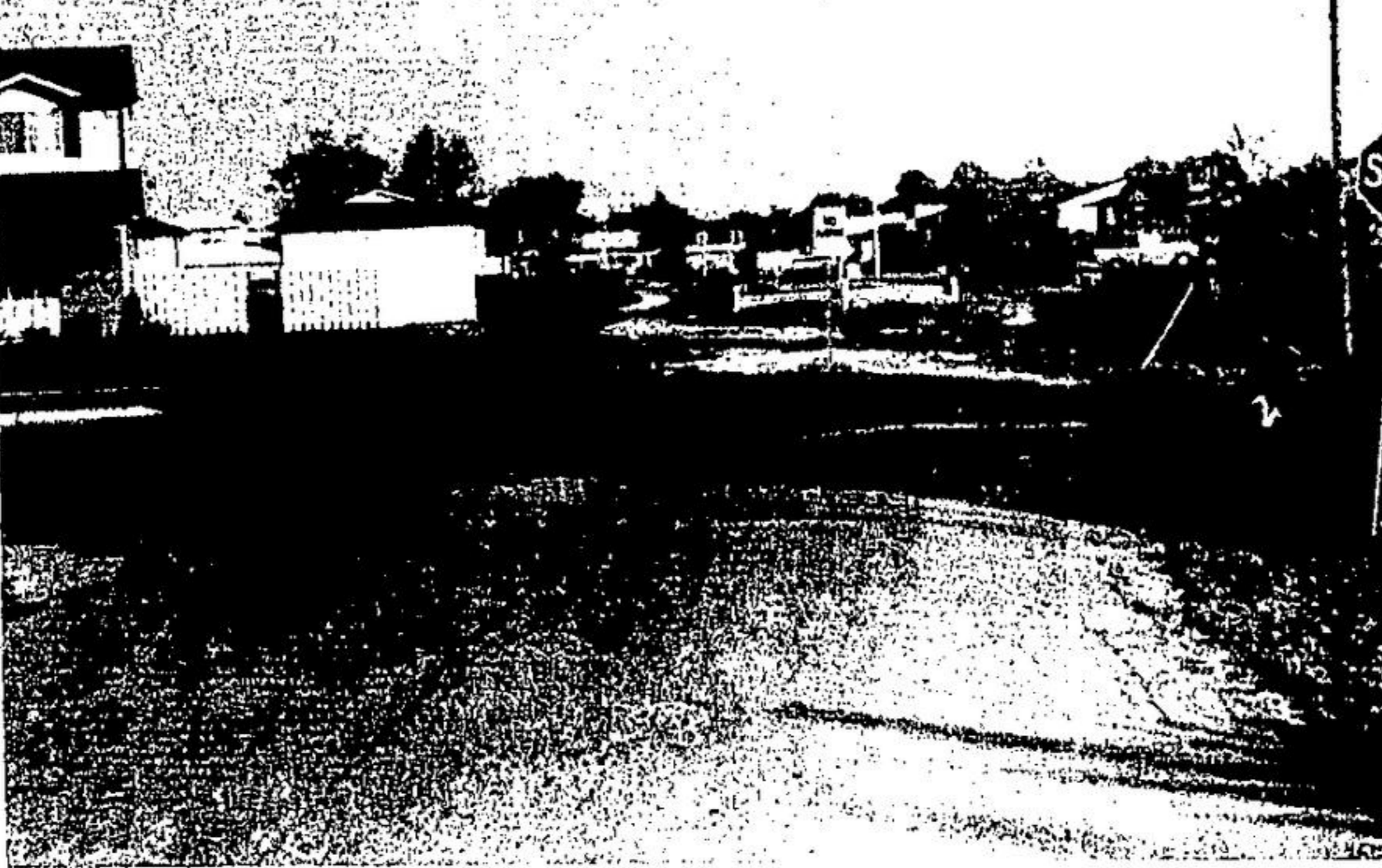
EVER WONDER, when you drive through town, why Division St. doesn't go through? At this corner Warren Grove and Bovis subdivision meet and this untidy little patch of ground and a barricade prevent through traffic. "No dumping" says the sign, somewhat irreverently.
