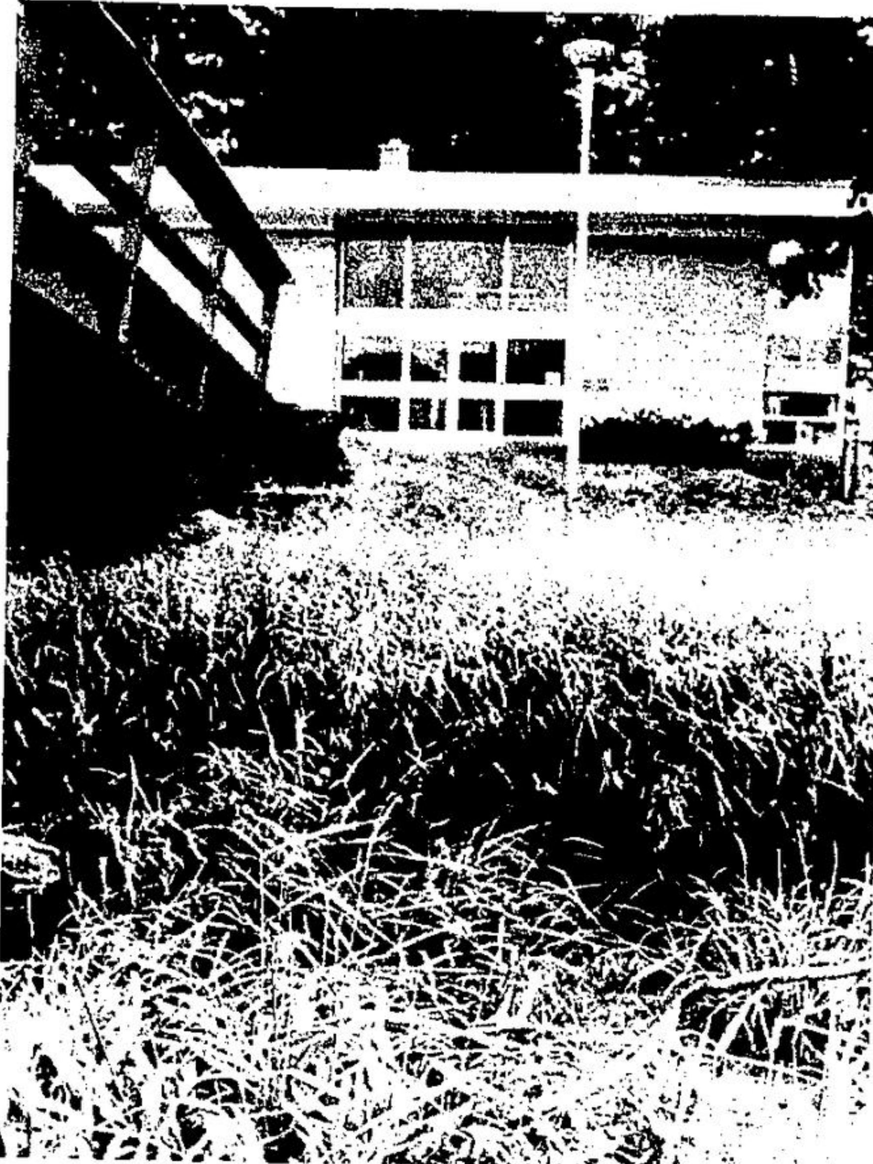
LIBRARY BOARD MEMBER NORM Elliott complained to the board last Wednesday about the overgrown state of the weeds in School Creek. Some of them were four feet high, he said. Mr. Elliott called for a permanent solution to the annual problem. Two days later town men cut down many of the weeds.
