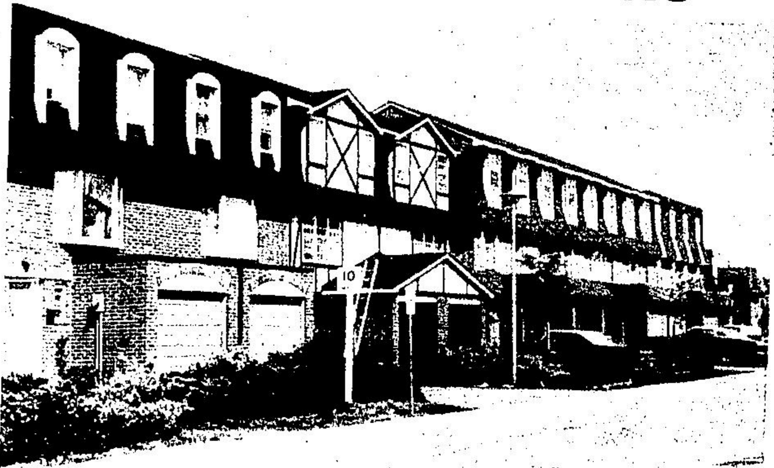
ministry established the Ontario Residential Condominium Study Group in November of 1976 to make recommendations. This group met with condominium
